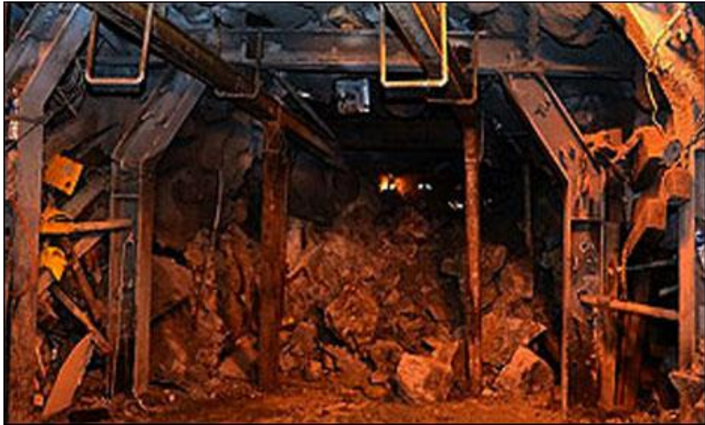
Figure 1.3: A collapsed mine tunnel. Adapted from [12]
