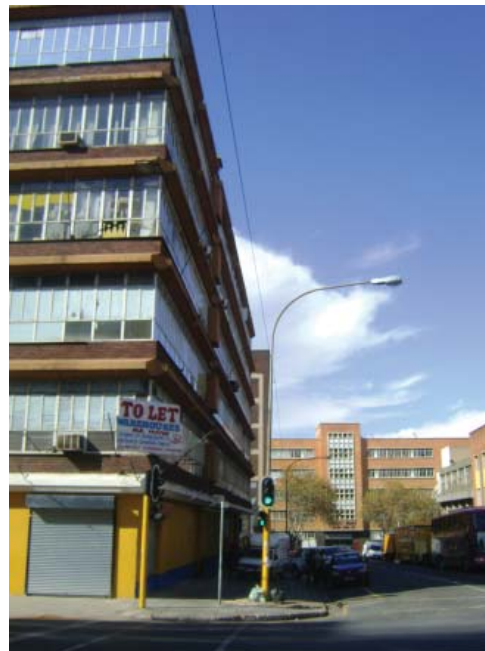
Fig 4.4b, newly renovated building to let
