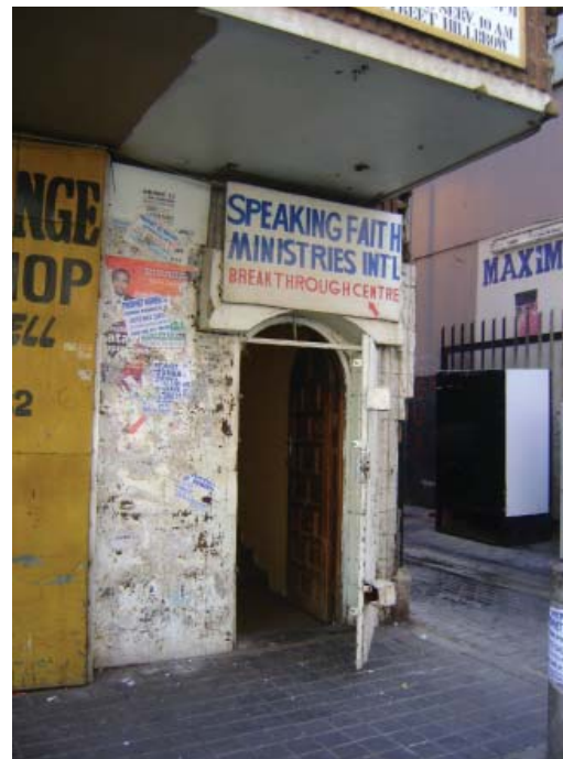
Fig 3.39b, Narrow main entrance into the church
