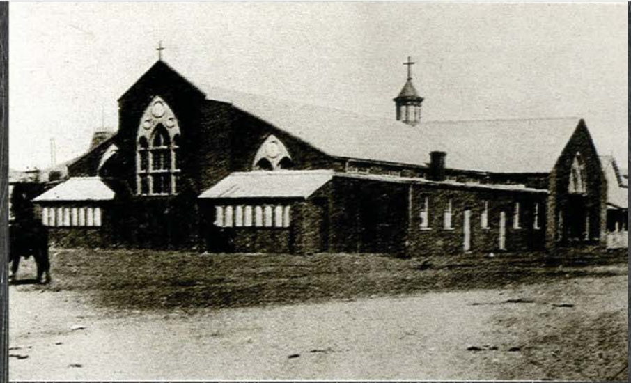
fig 2.4, St Mary's Church Building, (van der Waal 1986:14)
