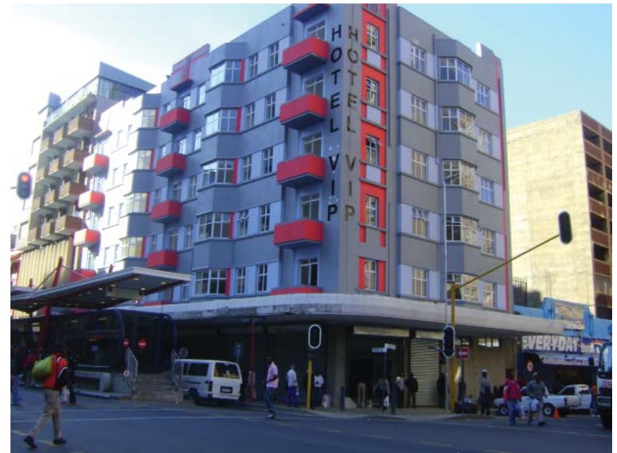
Fig 4.4c, newly renovated building ready for occupation as a Hotel
