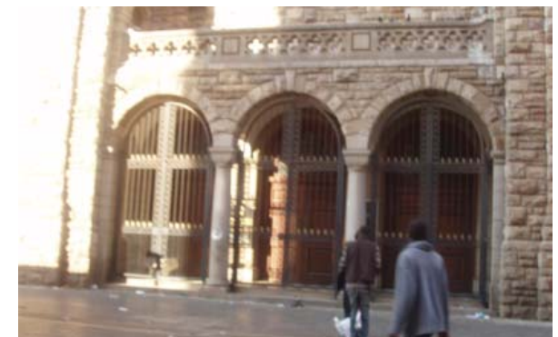
Fig 3.31, CCSMV, locked access
