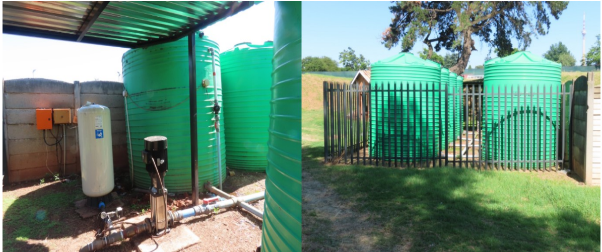
Figure 10: White elephant boreholes not in use or connected to a water storage system (Rodney Matentshi, 2020).
