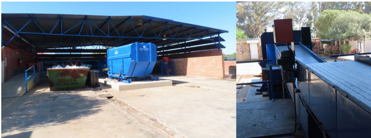
Figure 13: Colour coded waste stationed at west campus student's residence (Rodney Matentshi, 2020).
