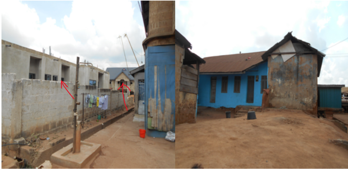
Figure 5.6: New buildings (arrowed in left picture) with modern styles replacing the typical compound housing type on the right inside the grid of Abuakwa, December 2019.
