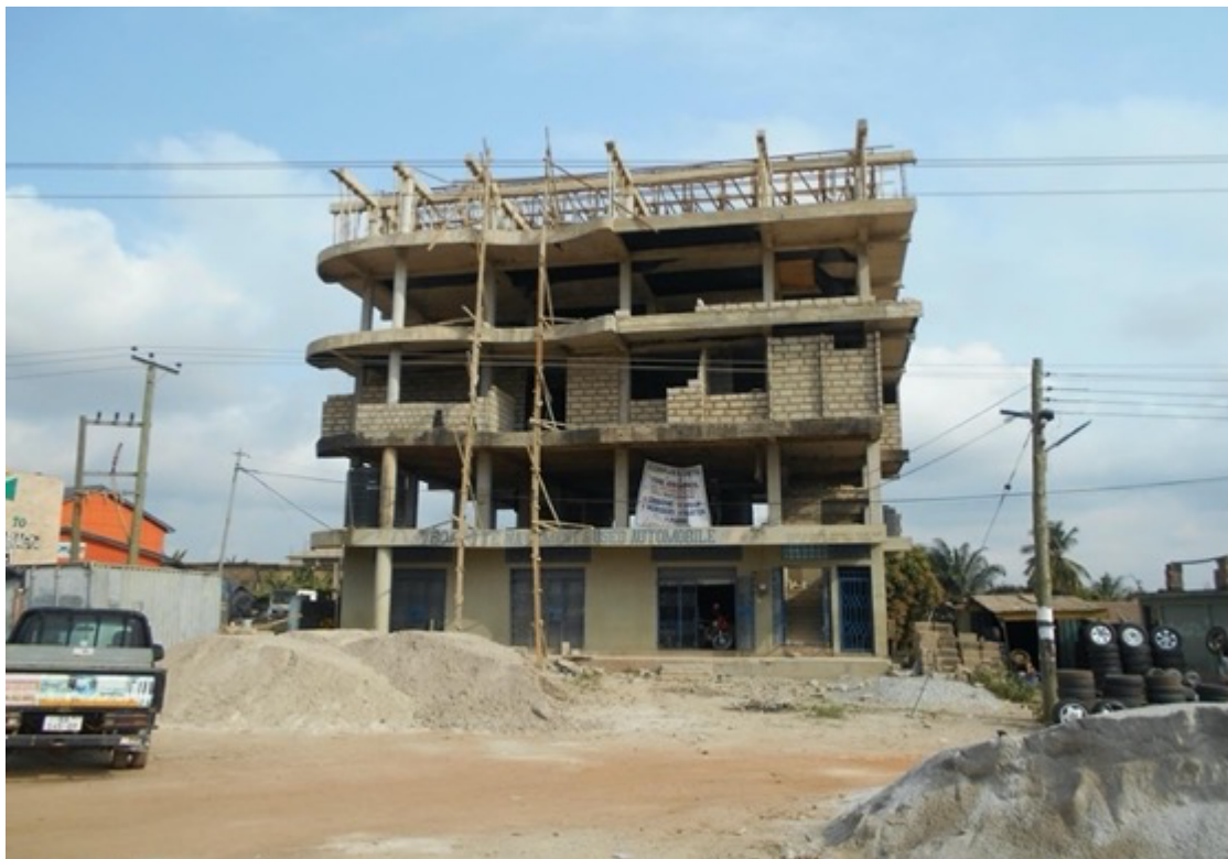
Figure 5.11: A building under construction showing verticalisation in the core area of Abuakwa, December 2019
