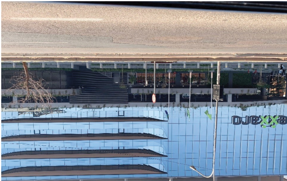
Figure 92_ New Building with non-active frontage (Author-2019)
