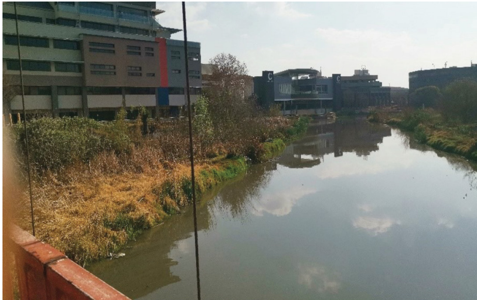
Figure 134_ pedestrian bridge over Hennops river (Author-2019)
