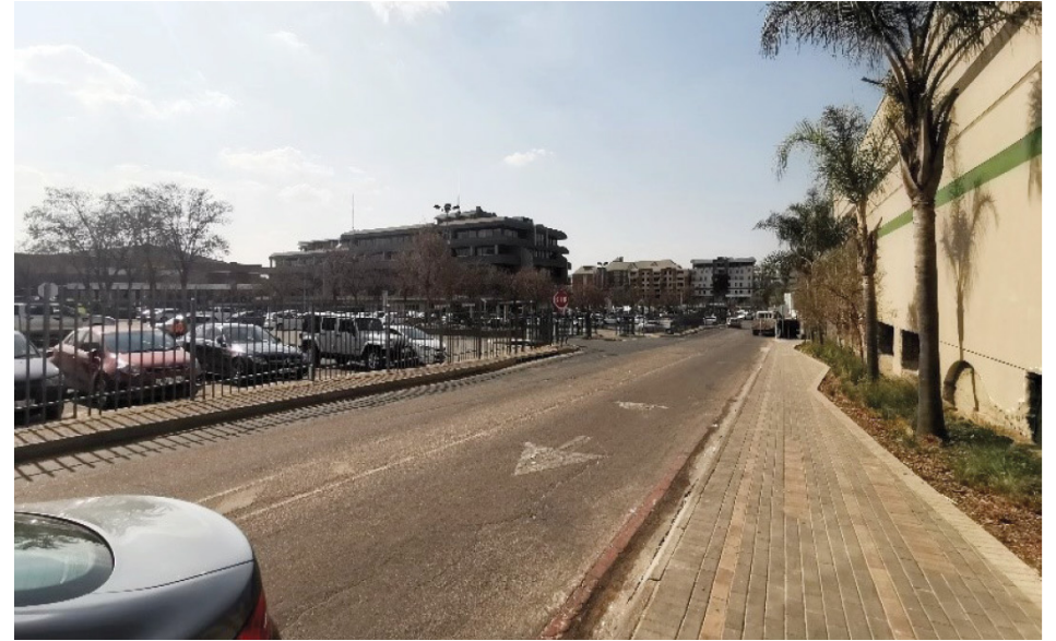
Figure 121_ Narrow (1.8mtrs) and inactive sidewalk along Gordon Hood Rd (Author-2019)
