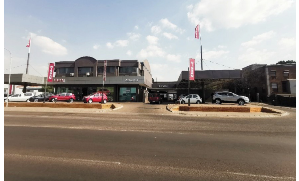
Figure 125_ Non-active fronts on Lenchen Ave (Author-2019)
