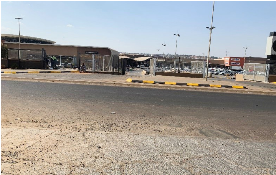
Figure 68_ Poor state of roads infrastructure (Author-2019)
