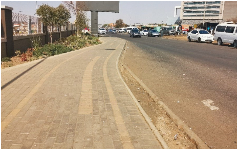
Figure 114_ Inactive paved pedestrian sidewalk (Author-2019)
