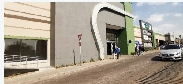
Figure 22_ Non-active sidewalks (Picture by Author)
