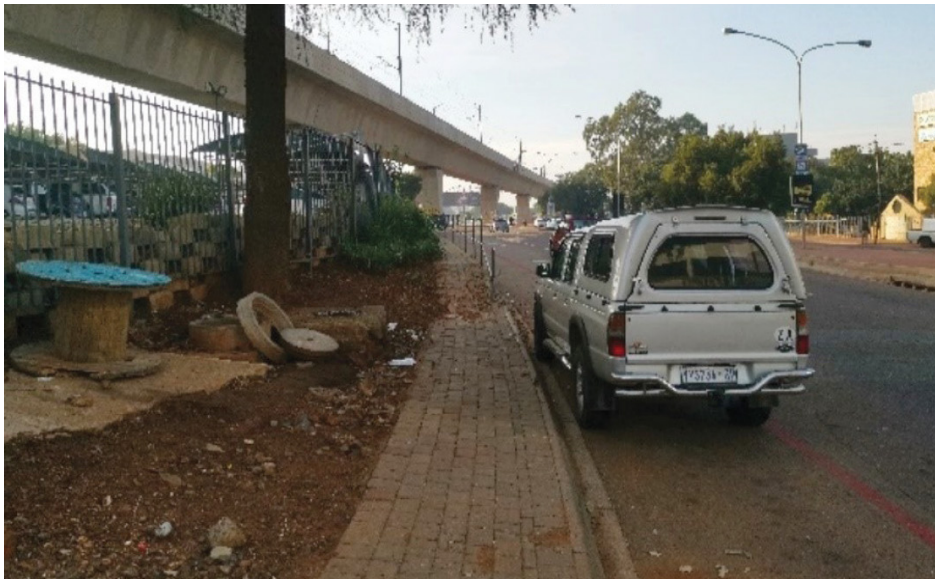
Figure 96_ Narrow sidewalk (1.5 mtrs) along West Avenue (Author-2019)
