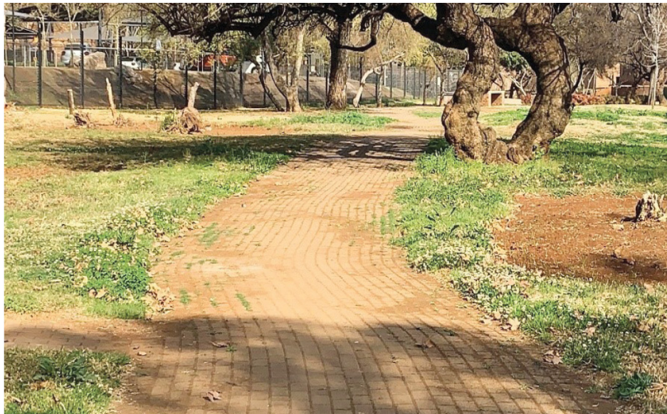
Figure 84_ Disused park infrastructure (Author-2019)
