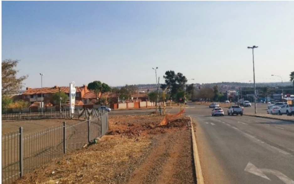
Figure 148_ Main Pedestrian feeder route from Metrorail on Gerhard St (Author-2019)
