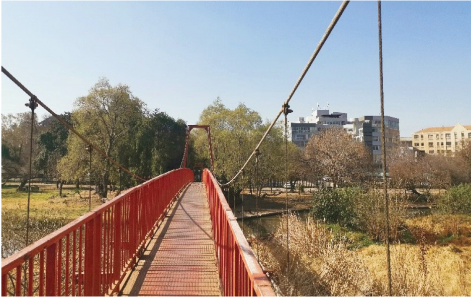
Figure 136_ Pedestrian Bridge over Hennops river (Author-2019)
