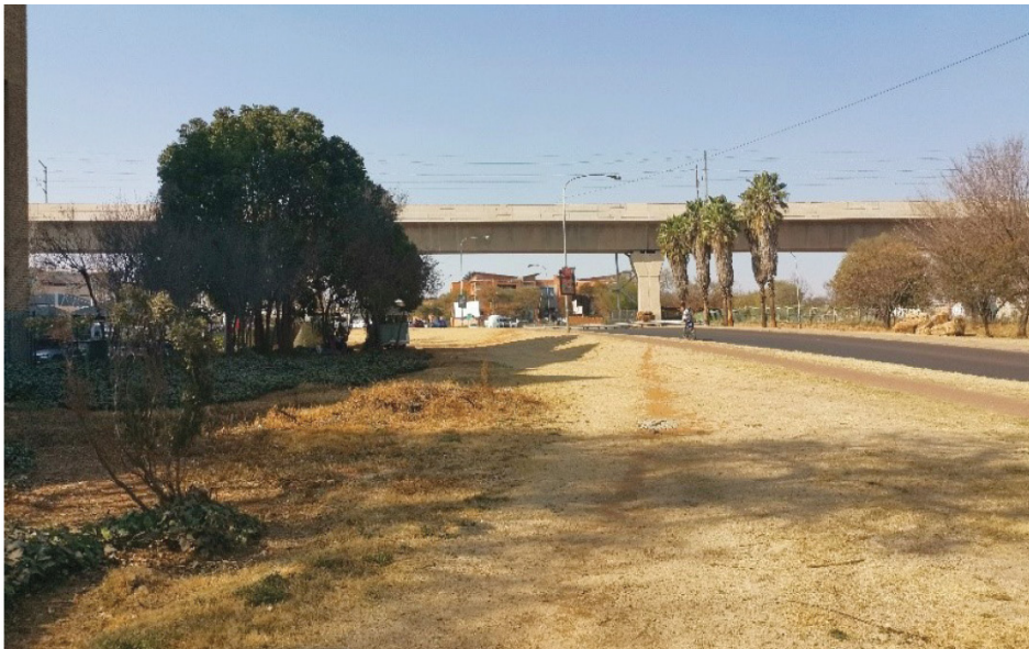
Figure 138_ Lack of NMT infrastructure on Lenchen Ave (Author-2019)
