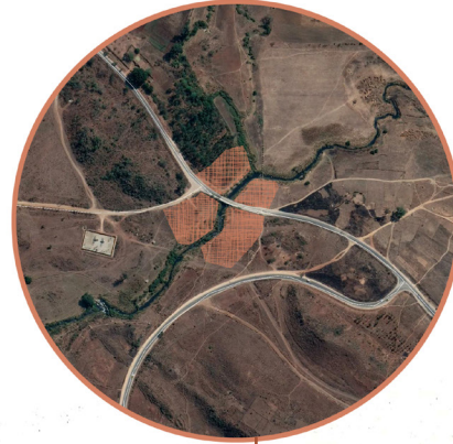
Site Context: Feruka Bridge
