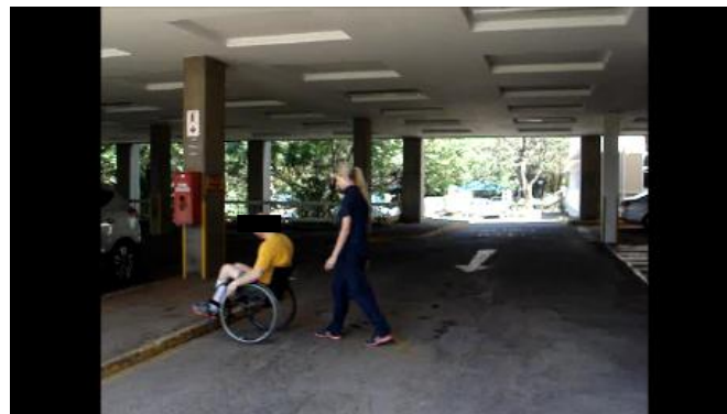
Photograph 3.10 Low curb (Measured to be 10 cm as required)
