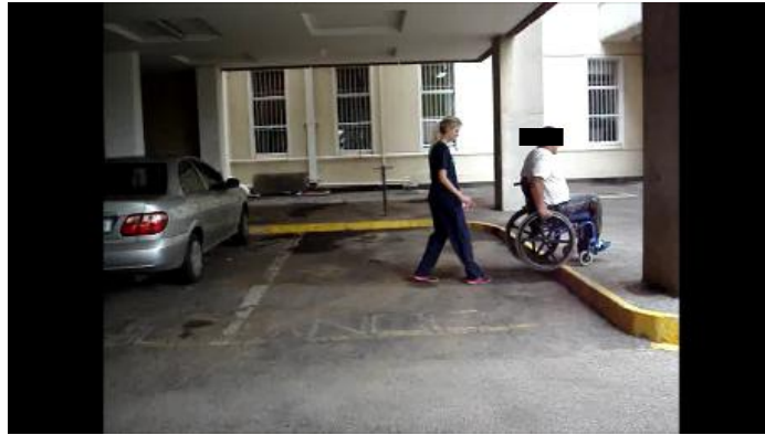
Photograph 3.11 High curb (Measured to be 15 cm as required)
