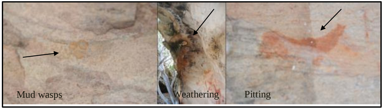
Figure 13: Factors causing deterioration at BKS 09, Cederberg [Photos by Elijah Katsetse: 2014]
