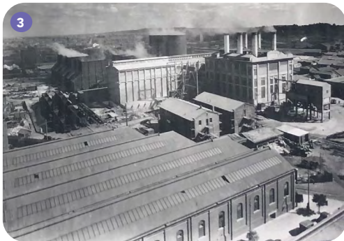
Fig 7.14: Jeppe Street Power Station 1930 looking west (Source: Museum Africa)
