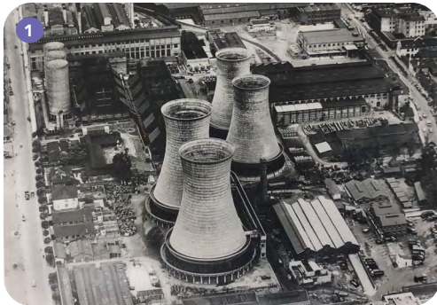
Fig 7.12: Aerial view of power precinct 1956 looking east (Source: Museum Africa)
