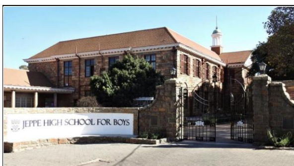
Figure 7: Improvement and Restoration of the main Gate (Dickie Fritz Gates).
