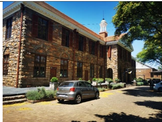
Figure 9: Façade of Jeppes Main Hall Building Condition
