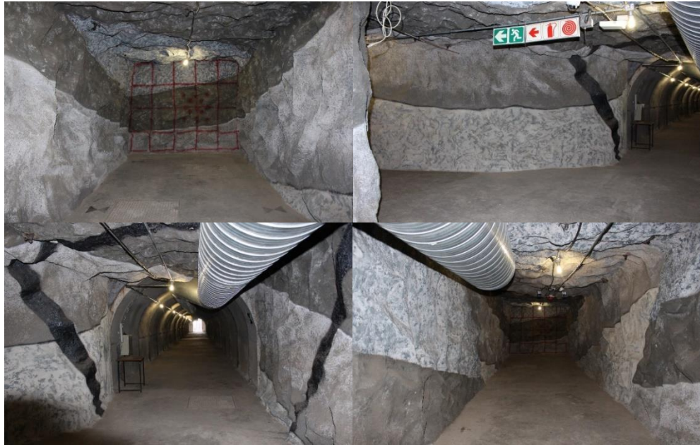
Figure 4.11 Wits Mockup-mine (Source: Author)
