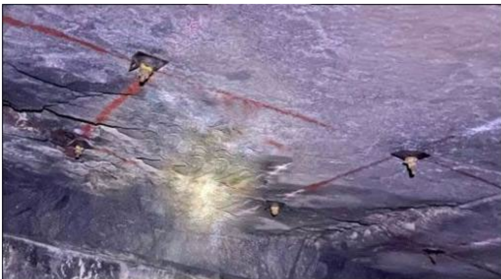
Figure 1-3: Resin bolts installed underground.
