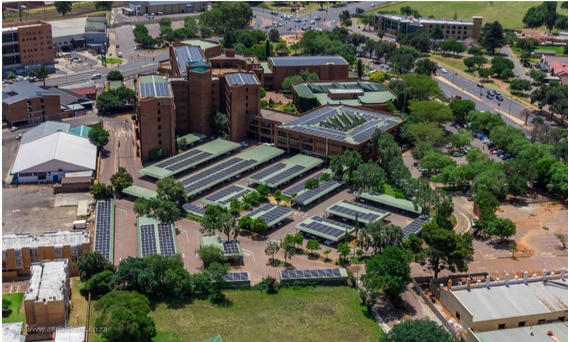
Figure 4.1: Kempton Park Civic Centre Solar PV (Source, Field observation, October 2019)
