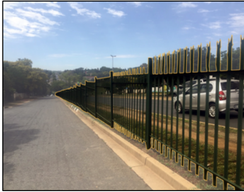
Figure 5.4 Fences between Bordeaux Drive and Jan Smuts Avenue (photograph by the author, 12/11/19).
