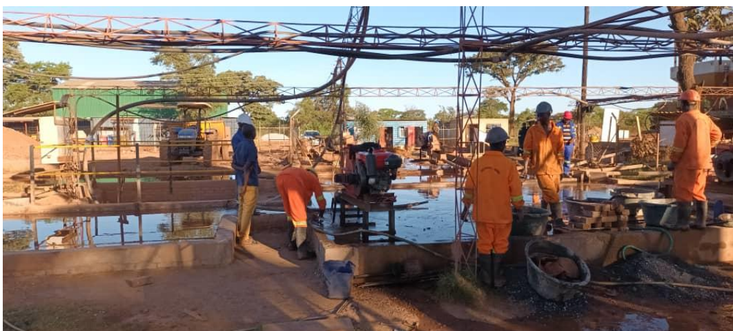
Figure B11 Picture of the panning bay
