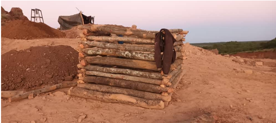
Figure B3 Picture of timber sets for shaft support
