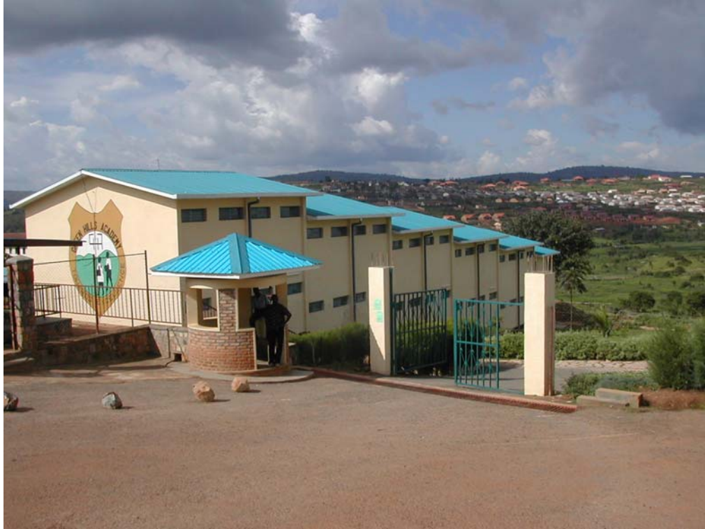
Figure 6. The boarding facility - this large roof area is still unutilized for rain water collection.
