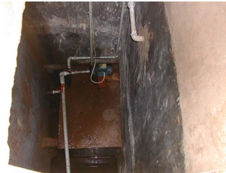
Picture 15. The pumping sump adjacent to the storage tank
