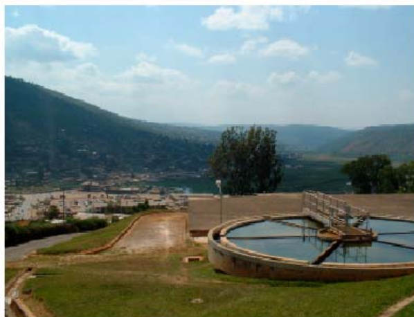
Figure 2.6 Electrogaz Purification Works
