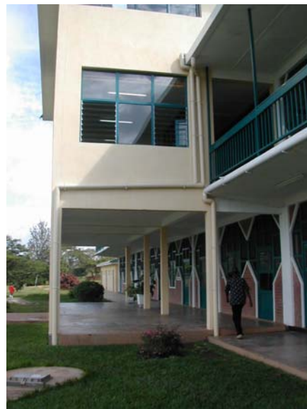
Picture 17. Neat piping from gutters to underground tank.
