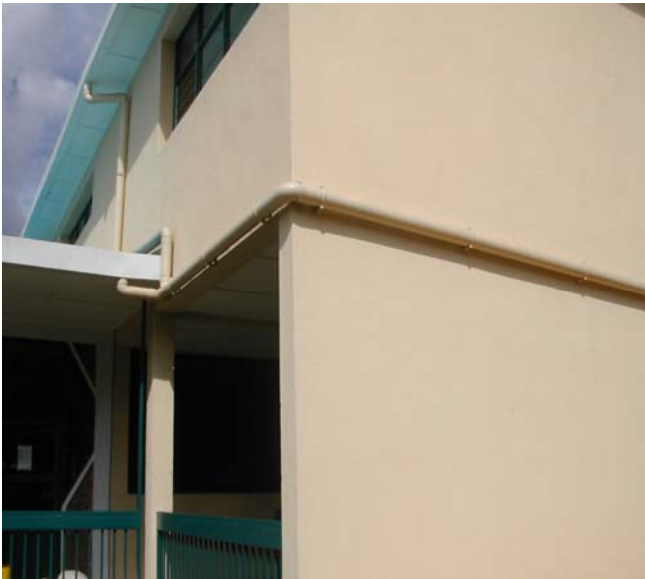
Picture 17. Neat piping from gutters to underground tank.
