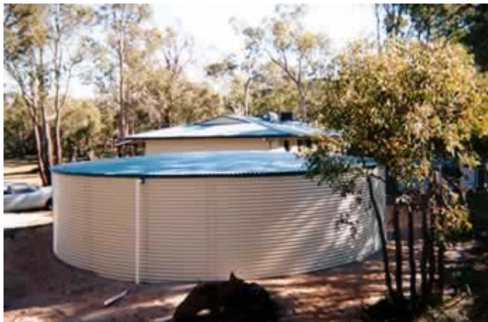
Figure 3.9 Large Corrugated Steel Tank In Australia
