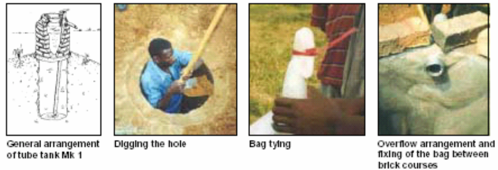
Figure 3.12 Sleeve Wells
