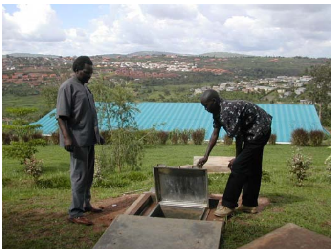
Picture 13 Mr. Ainea Kimaro and the school technician inspect the underground storage tank
