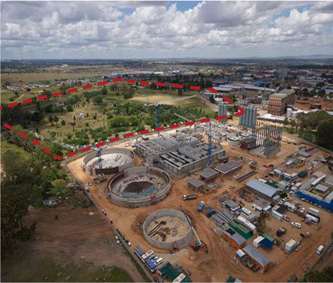
Figure 4.18 The Treatment Plant (SAME Water, 2014) The current state of the proposed site is primarily abandoned with unconstrained vegetation.
