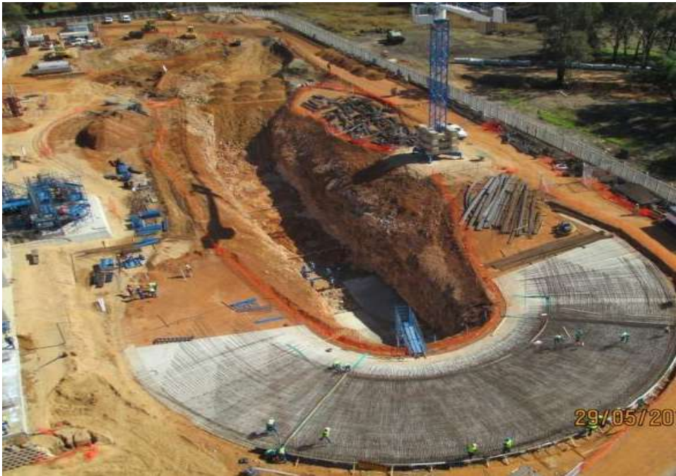
Figure 4.11 Treatment Plant Site Photographs, (TCTA, 2008) The site construction photos showcase the thick concrete construction used to contain the basins. The major materials used are reinforced concrete and steel structures. The steel is primarily used to create walkways above the basins.
