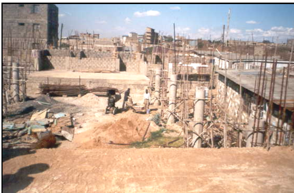
Photo 5.7. Concrete columns in a low-income construction in Dandora.
