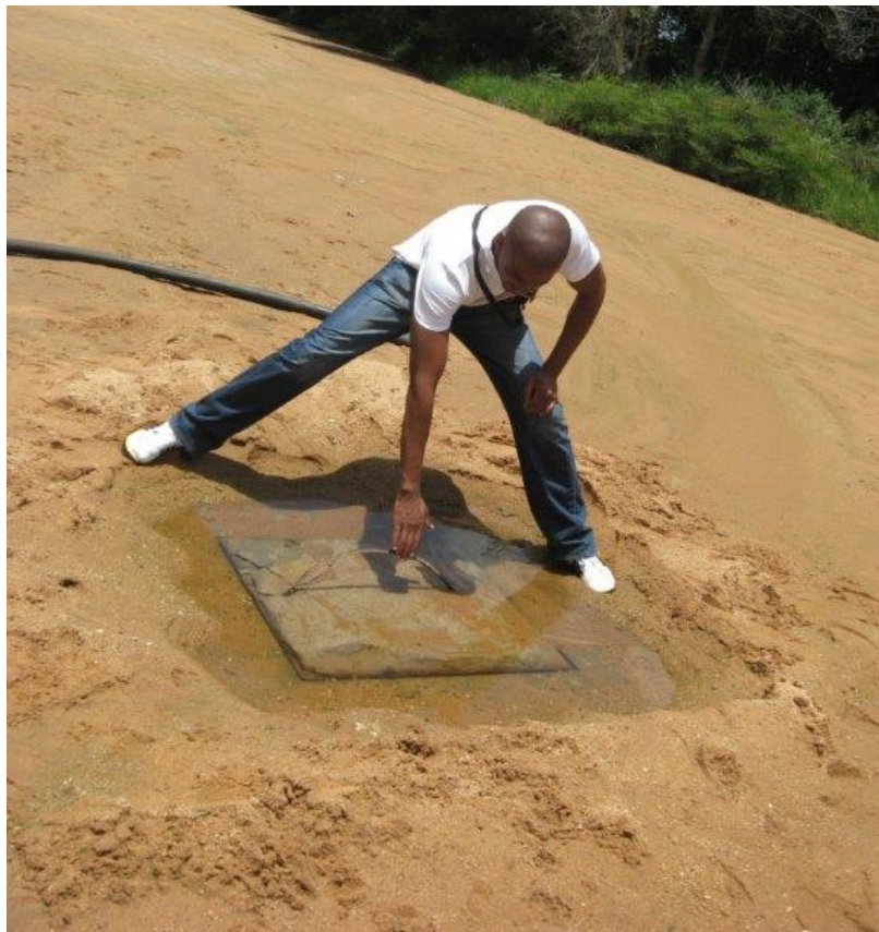
Figure D 12: Sump constructed for water pumping
