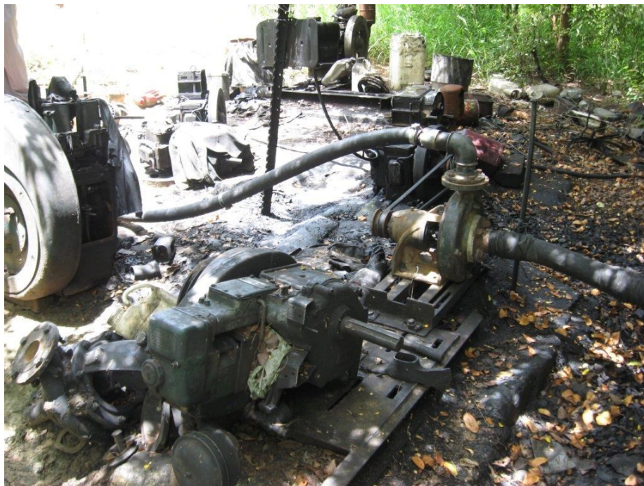
Figure D 10: Pumping station from the river
