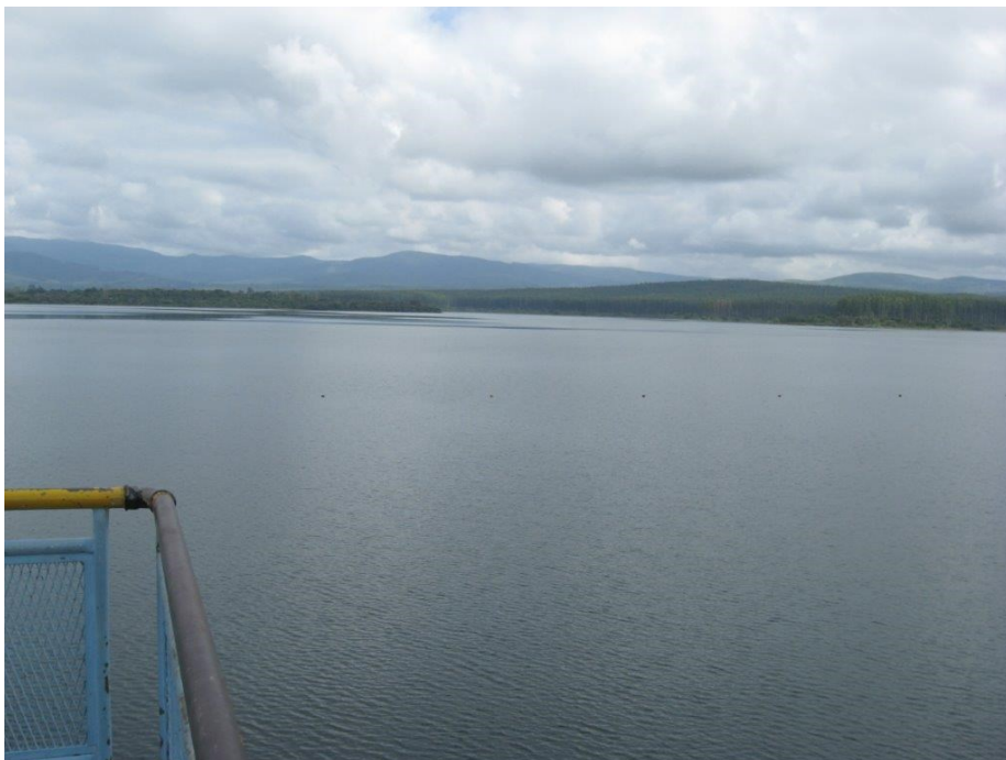
Figure D 14: Tzaneen dam
