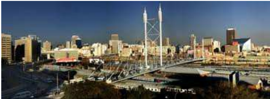
Fig.3 Mandela Bridge, source: google
