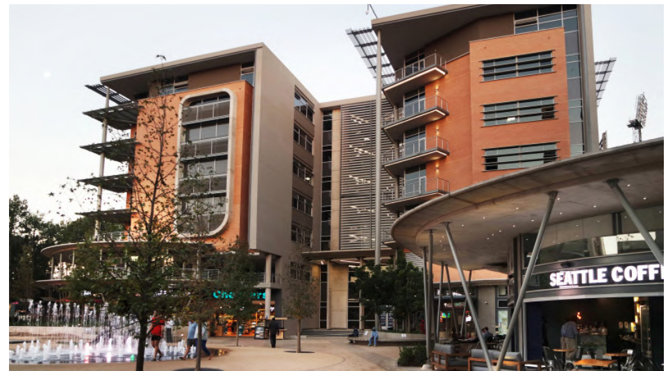
Figure 5. 20: Image showing Loftus Park retail entrance (Sefolo, 2018)
