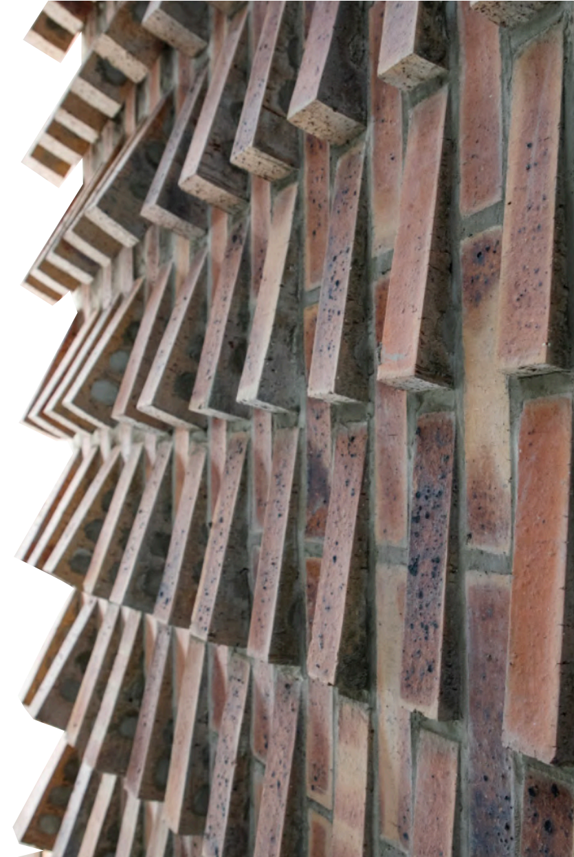
Figure 9.24: Image of textured brick facade (mashabanerose, 2022)
