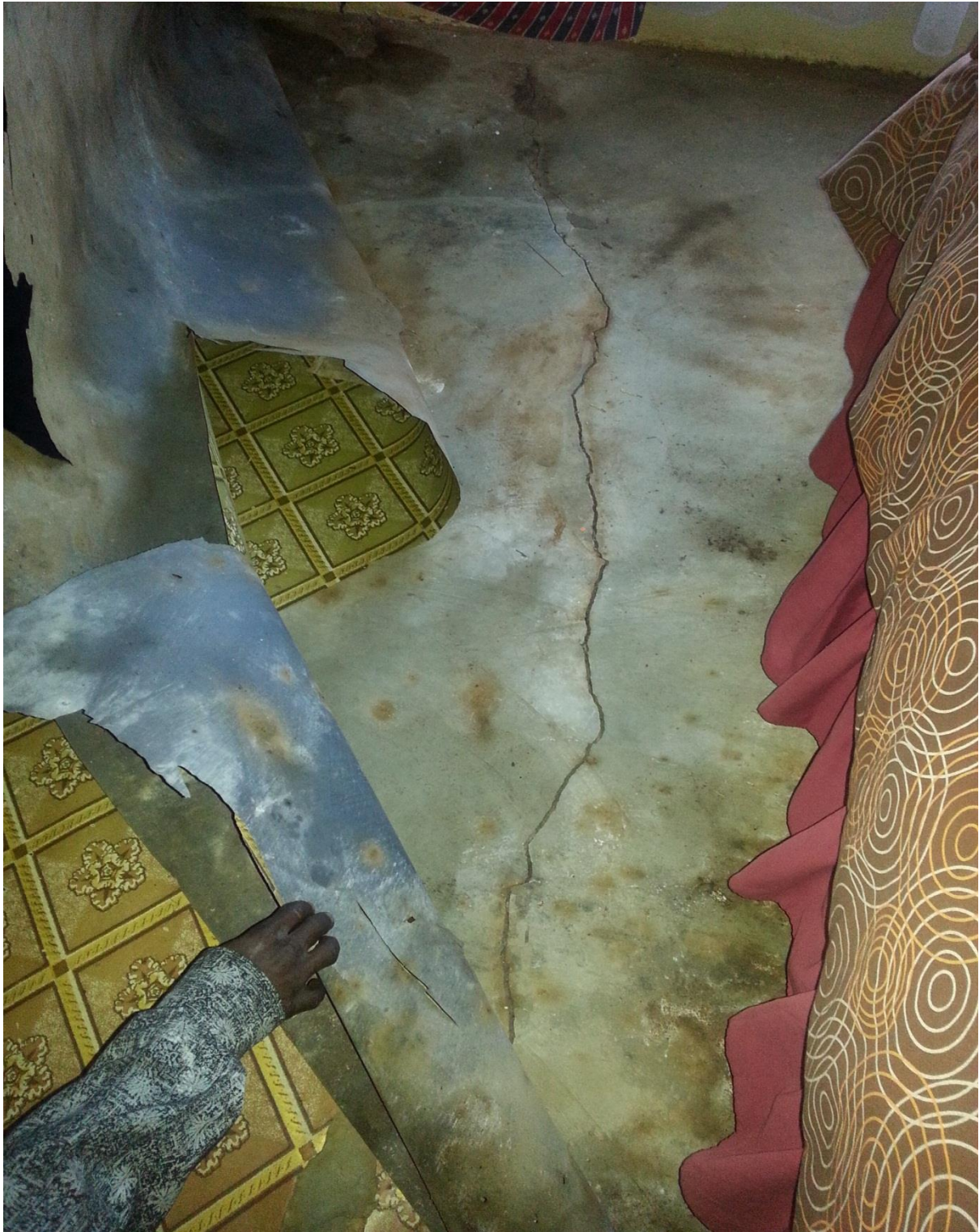
(Photo 3: A crack in the floor of the house as a result of sinkhole damage. Source: Kgopolo Makgopela; 2013)
