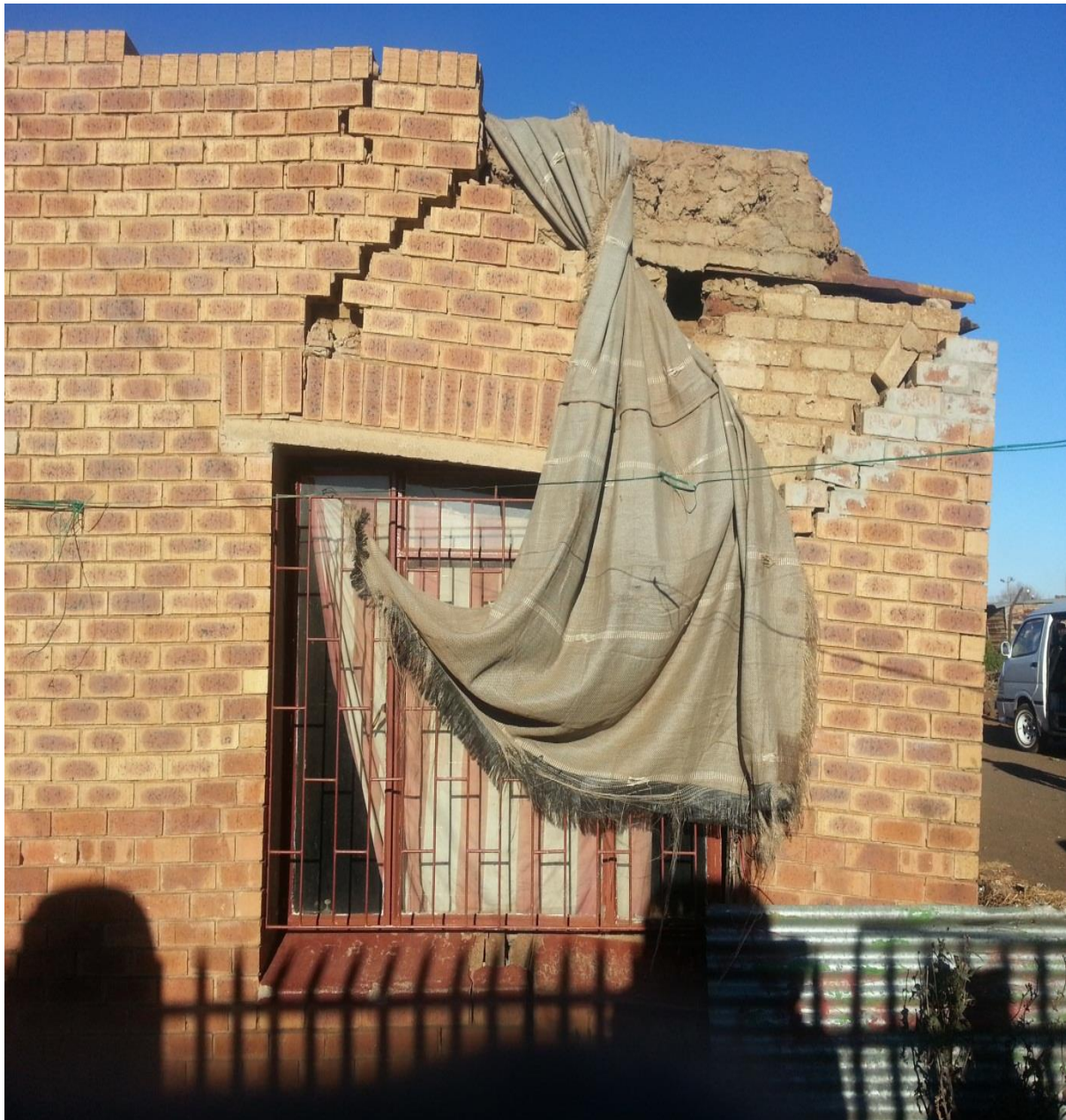
(Photo 2: The side of the house collapsing due to sinkhole. Source: Kgopolo Makgopela; 2013)
