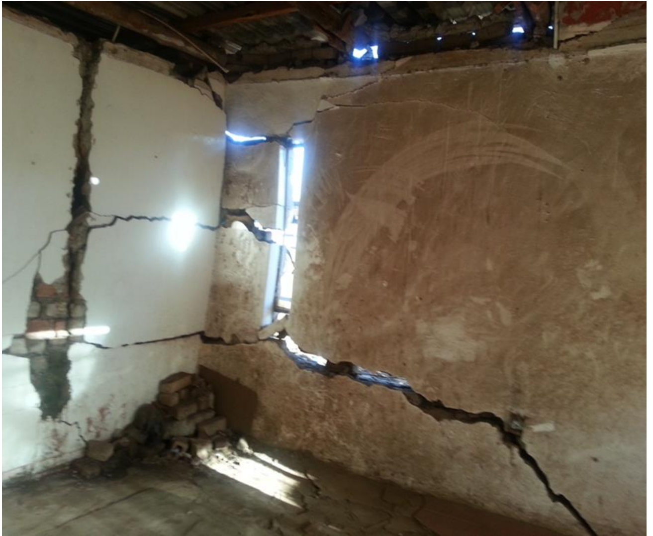
(Photo 1: House on a sinkhole with visible heavy damage to the walls, ceiling and floor. Source: Kgopolo Makgopela; 2013)
