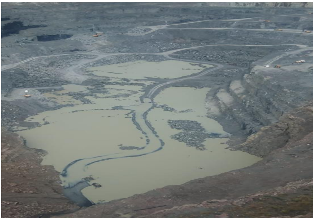
Figure 4-9: Flooded open pit bottom
