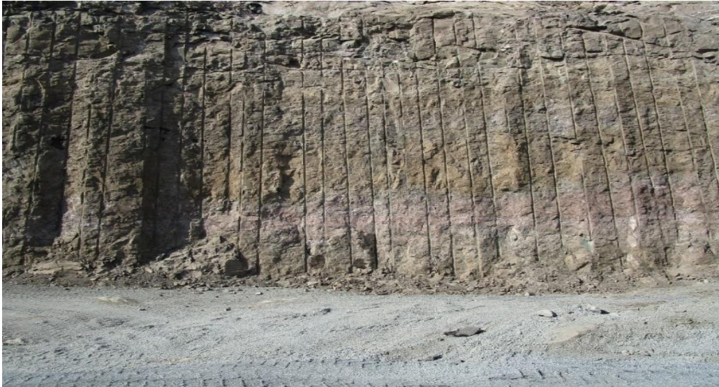
Figure 4-19: Exposed pre-split barrels from the high wall
