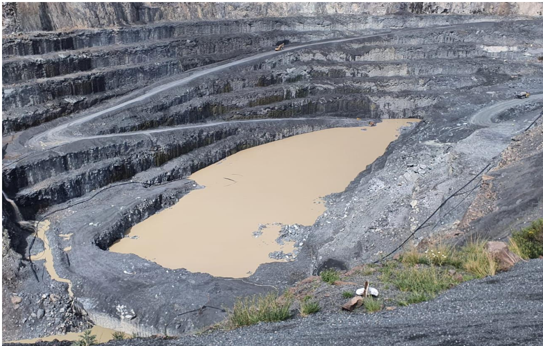
Figure 4-3: Pit flooding due to heavy rainfall
