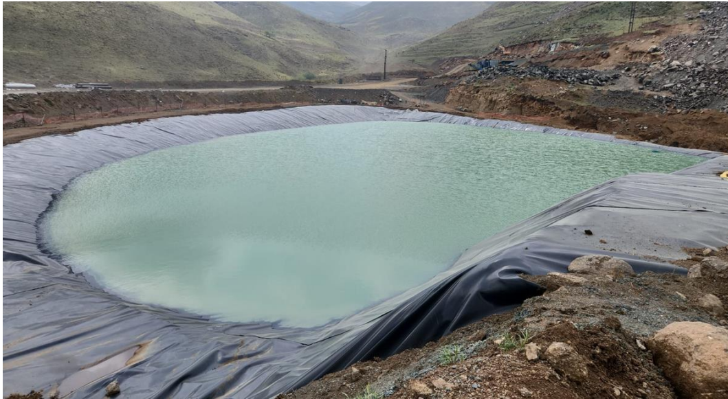
Figure 4-11: Flocculant dam
