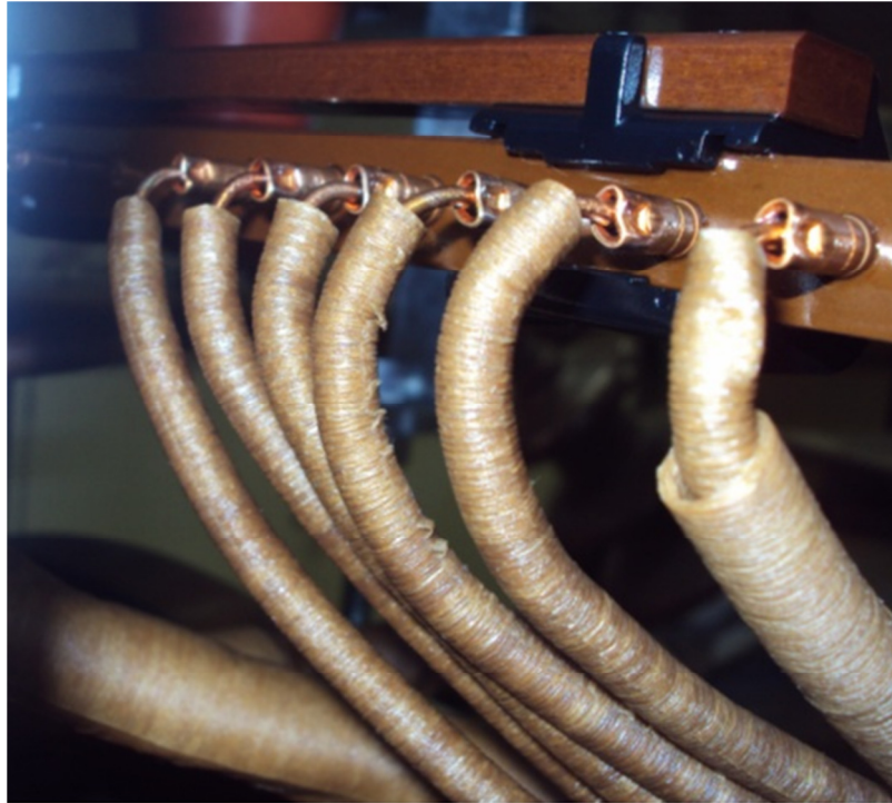
Figure 31: Copper windings connected to a tap changer
