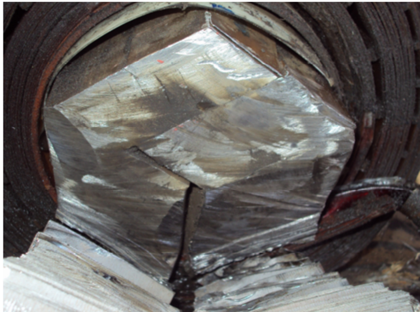
Figure 32: Cross sectional view of the Hexa-transformer core
