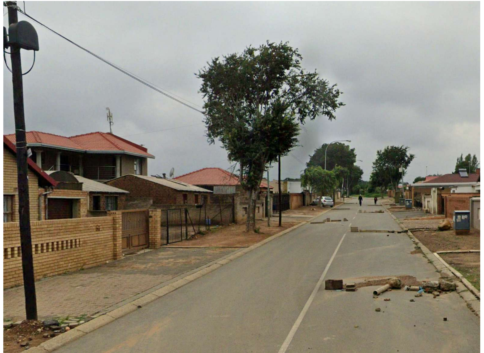
figure 67: Informal traffic calming measures in Soweto. (Author, 2022)
