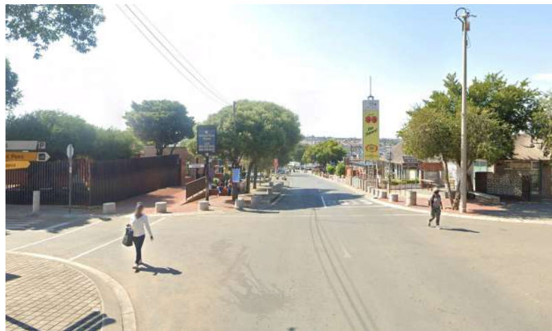
figure 93: Existing vilakazi street intersection. (Author, 2022)
