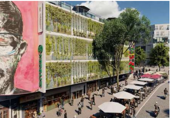
Sakhumzi restaurant upgrade
