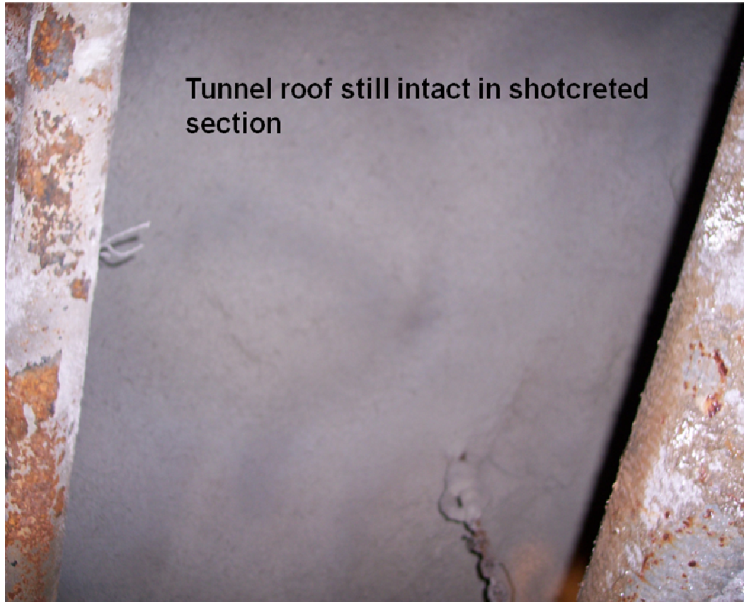
Figure 5.5c Close view of Mponeng Mine Level 109 shotcreted roof section (shotcreted roof section in Figure 5.5a) still intact and showing no signs of failure in the shotcrete as the shotcrete provides support through the beam support mechanism
