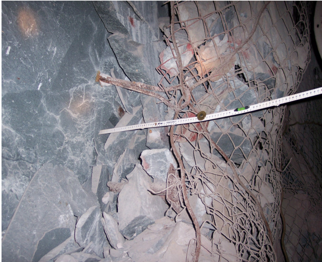
Figure 5.1c Side view of the loosened blocks (about 0.5m depth) held back by the mesh and lacing a few metres from the intact shotcreted section shown in Figure 5.1a and Figure 5.1b
