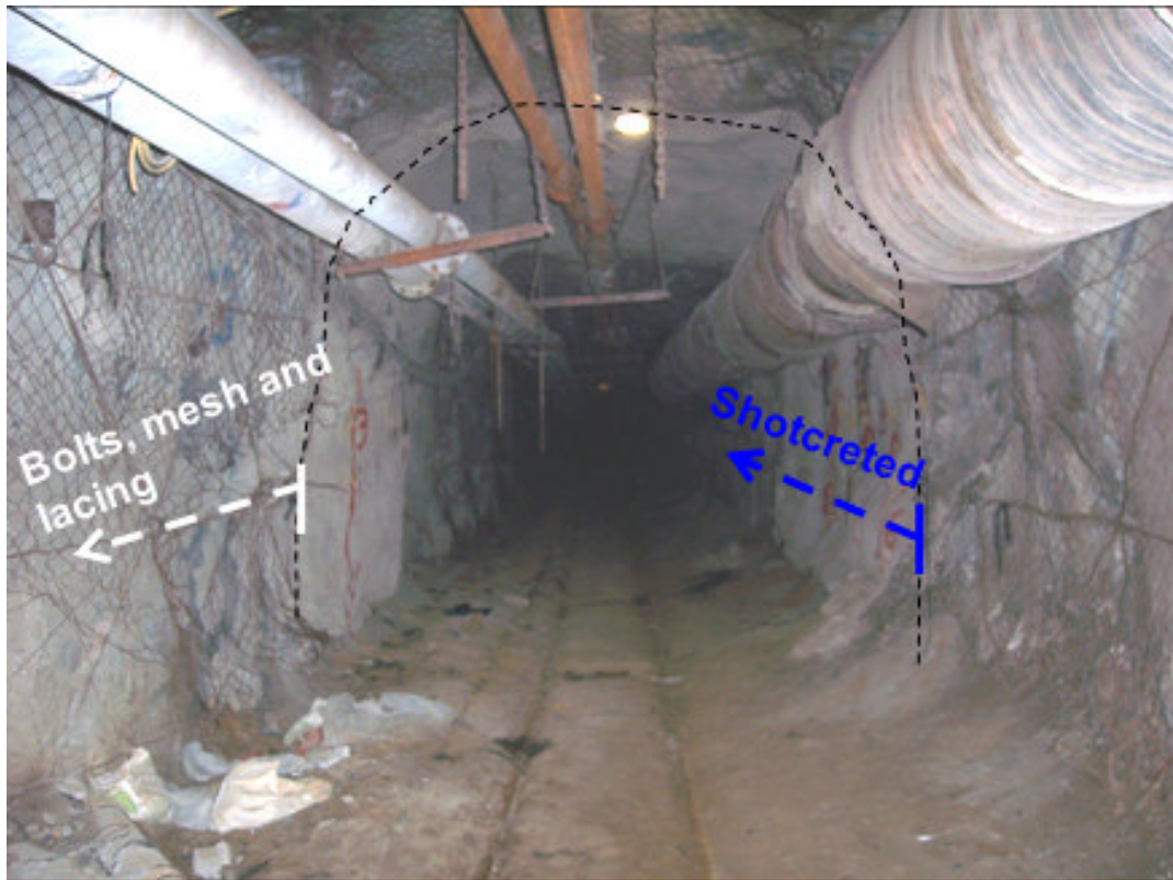
Figure 5.5a Demarcation between shotcrete, mesh and lacing support on Level 109 at Mponeng Mine. Shotcreted section shows no signs of loosening whereas the mesh and lacing section show signs of rock loosening.
