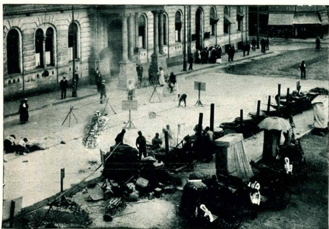
Photo of Asphalte Road being laid by Jenkins & Co., outside G.P.O., Johannesburg
