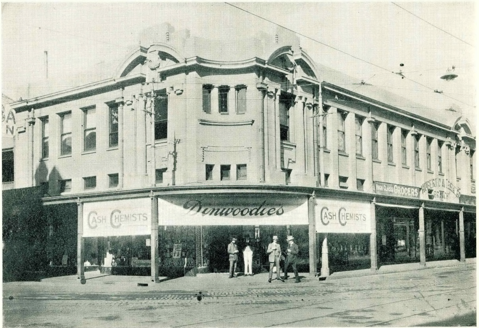
UNIVERSITY HOUSE, CORNER OF ELOFF AND PLEIN STREETS, JOHANNESBURG
