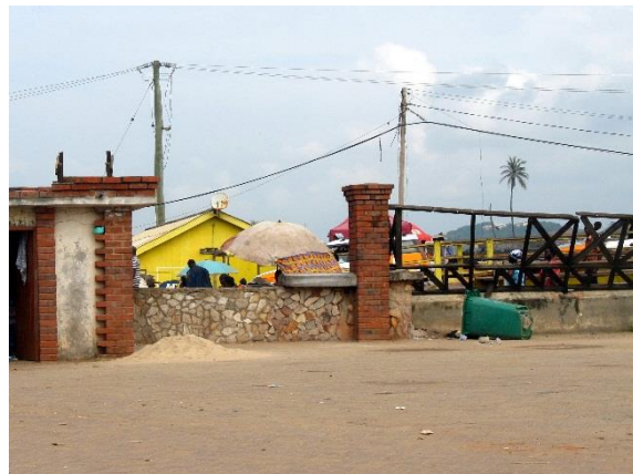
Figure 42. Bins for waste disposal at Lagoon Bridge
