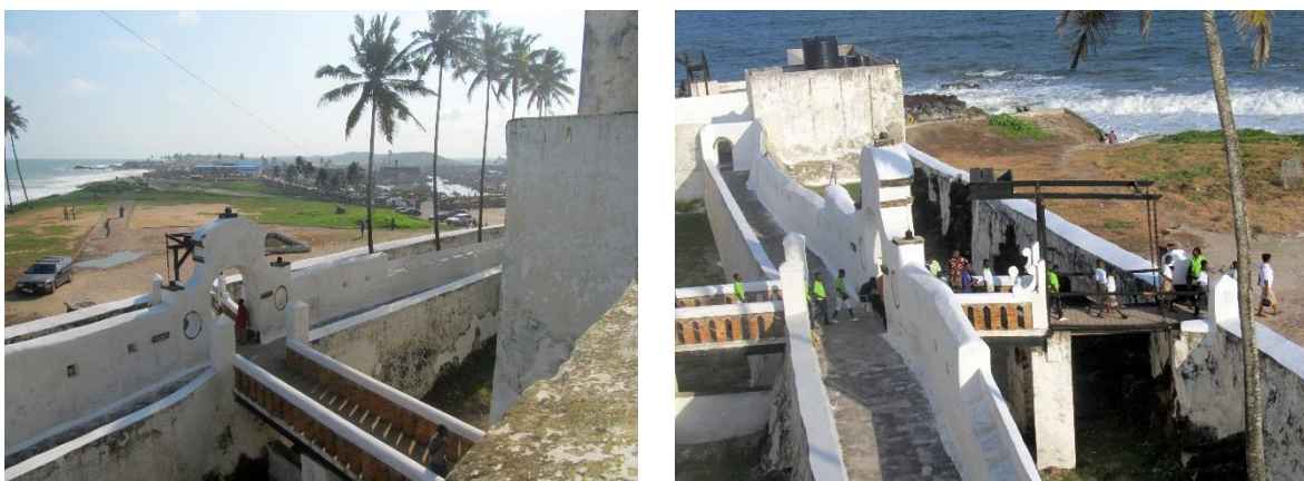
Figure 30. Entrance bridge to the Elmina Castle, repaired by the ECHMP
