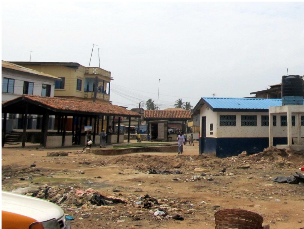
Figure 40. The proposed area for the arts and crafts market (initial constructions which were erected before the activity was stopped)
