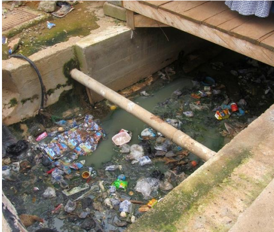
Figure 45. The new established drainage system in July 2012
