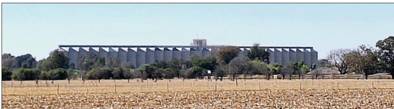
Figure 3: Sannieshof Grain Silo/Intake facility, North-West Province.
