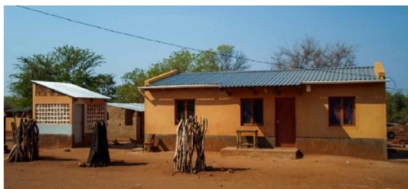
Figure 4 - Photo of a new house in the Benga Resettlement. Source: By Raquel Nobre (2017).
