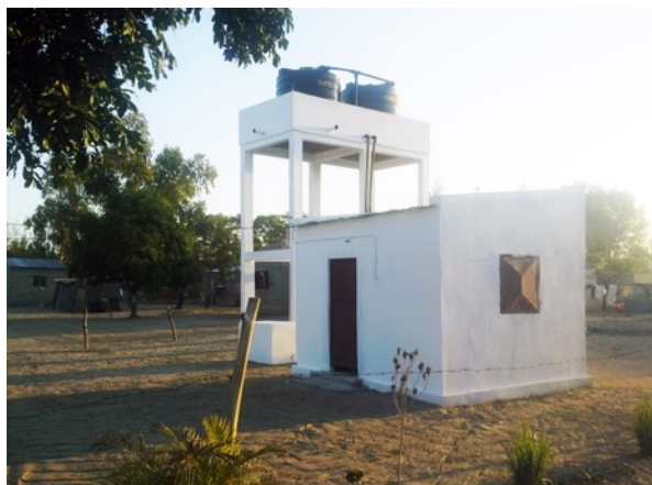
Figure 20 - Water supply system and the machinery room on the resettlement site. Source: CMM, 2016a.
