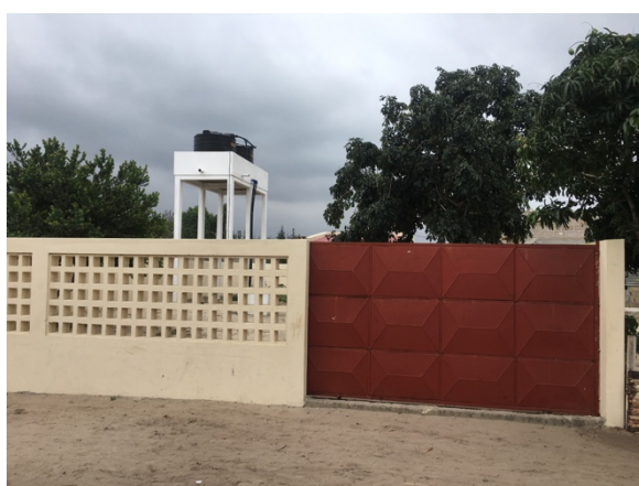
Figure 38 - Water tank and fence wall. Source: By author, October 2017
