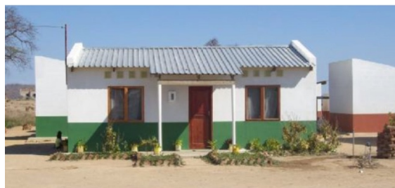
Figure 5 - Photo of a new house resettlement in Moatise. Source: Pedro (2011).
