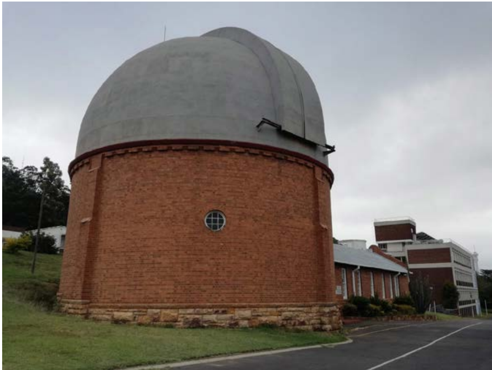
The Johannesburg Observatory. The building is made from red facebrick and the base of the building is the aforementioned orthoquartzite. The dome of the observatory is made from sheet metal, although the specific material is not discussed or mentioned.
