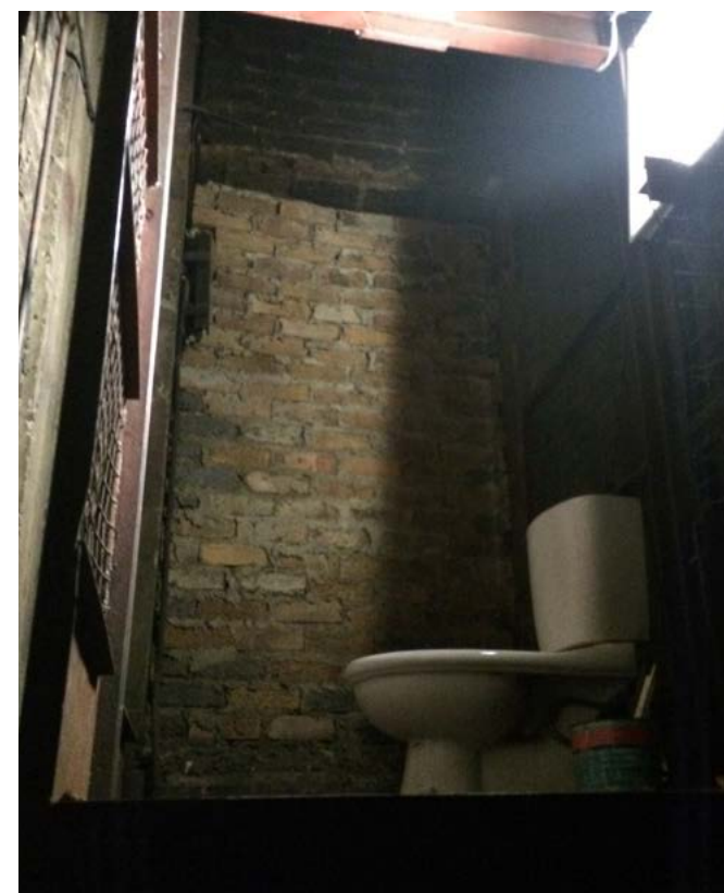
FIGURE 12: Toilet built in the old lift well
