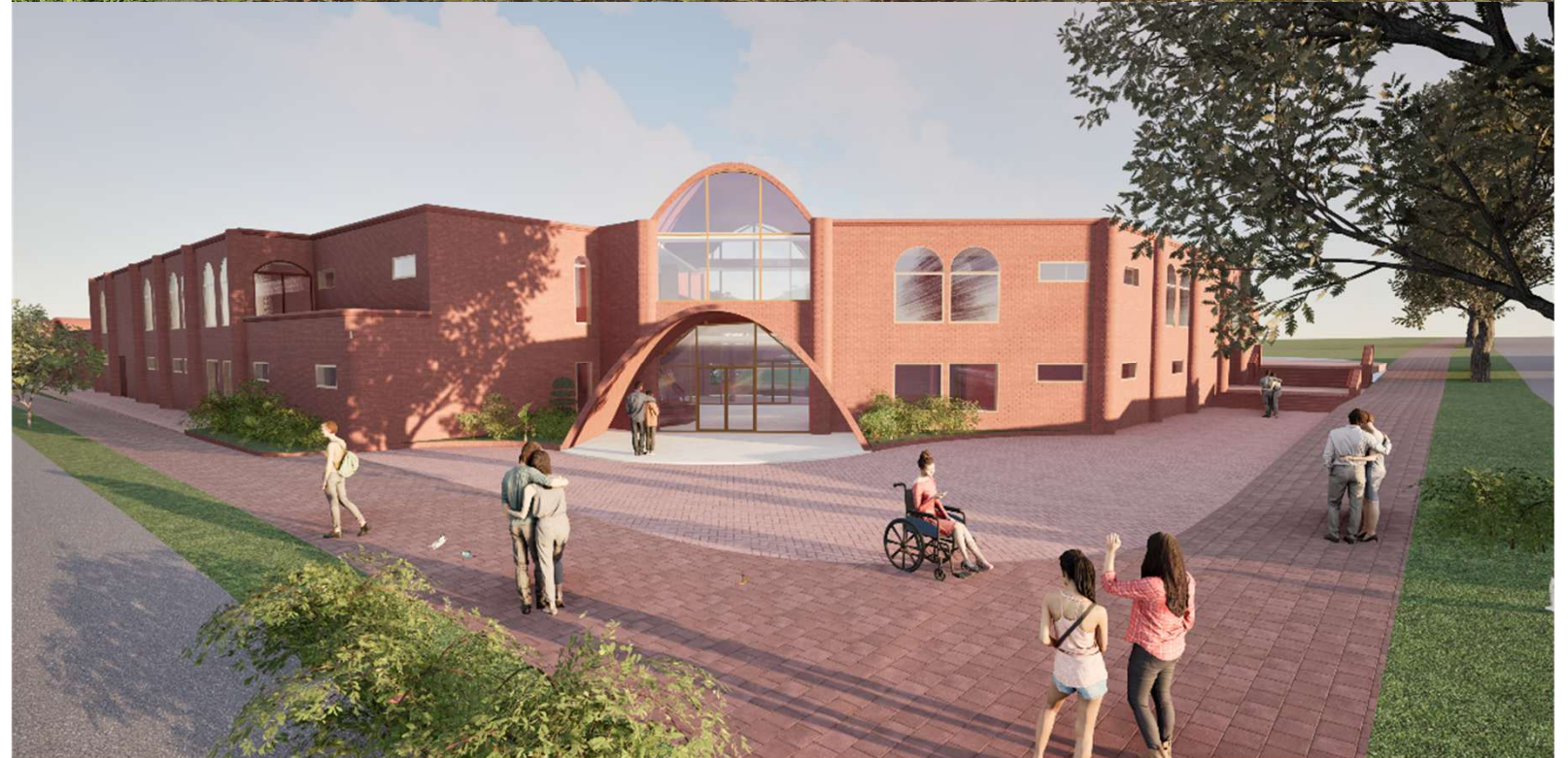
Figure 7.2: South-East Approach to Clinic Main Entrance
