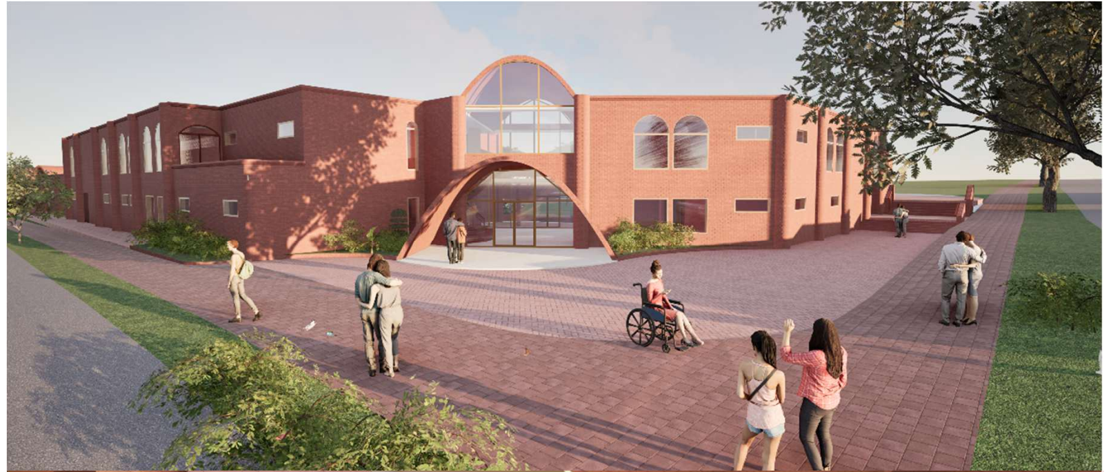
Figure 7.15: Main Entrance and Approach
