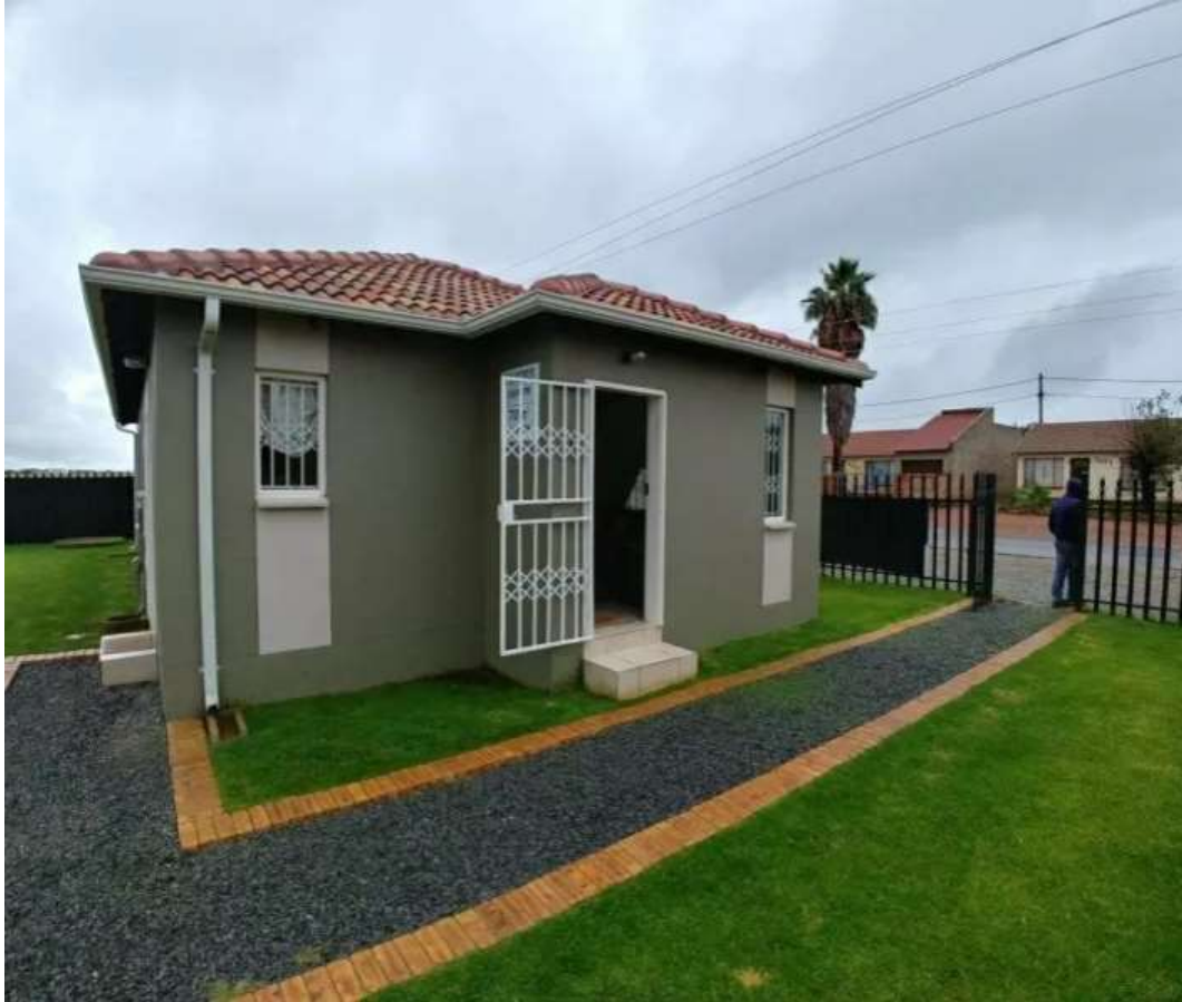
Figure 9: showing fenced off bonded house in Savanna City
