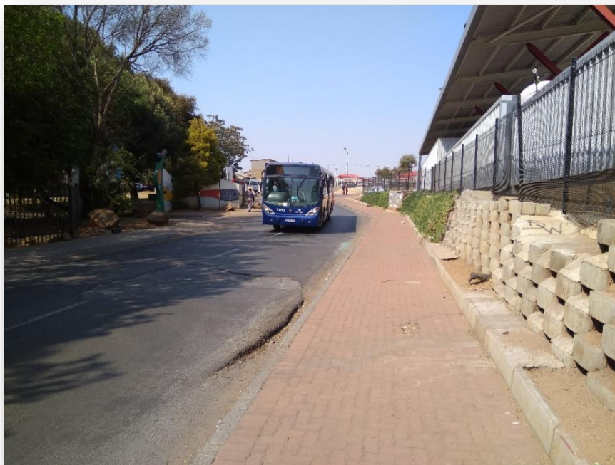
Photograph 10: Photograph showing Rea Vaya bus accessing the station from behind and not on Dmas/Mashinini road (Nduduzo Nyanda: 06/09/2017)
