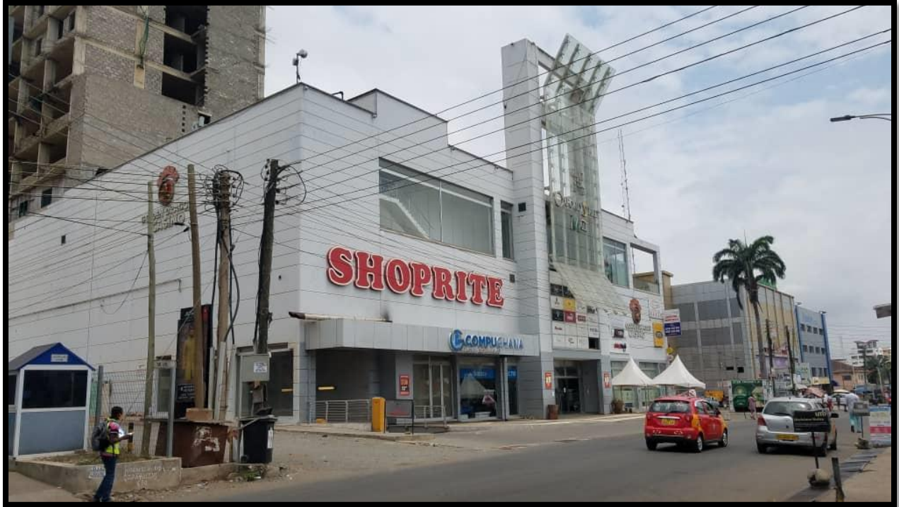
Photo 5.14: Electrical Lines Running Across Street (Photo by Lincoln Nyarko, 2020)
