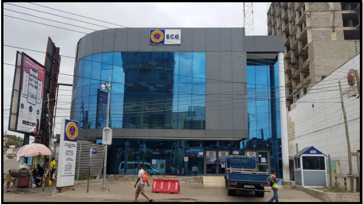
Photo 5.15: Electrical Lines Running Along Street (Photo by Lincoln Nyarko, 2020)
