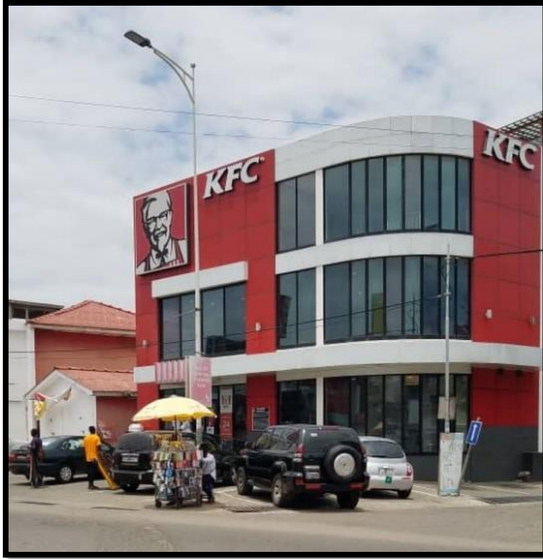
Photo 5.12: The use of Transparent Glass on the Ground Floor of KFC Restaurant (Photo by Lincoln Nyarko, 2020)
