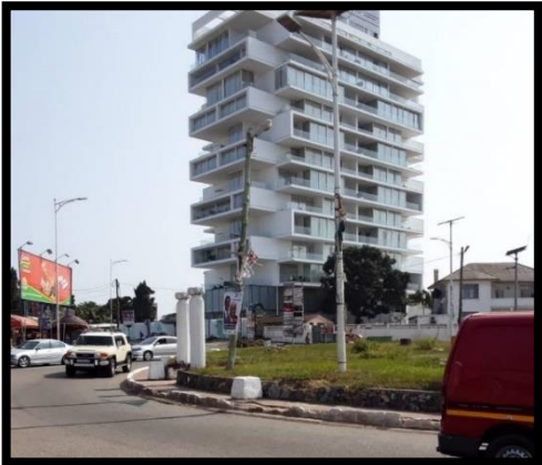
Photo 3.10: A Multi-Storey Mixed-Use Facility at Danquah Circle (Photo by Walter Ashong, 2020)
