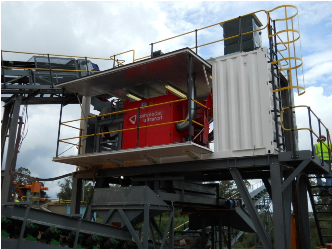
Figure 39. Containerised ROM optical sorter plant at CRG
