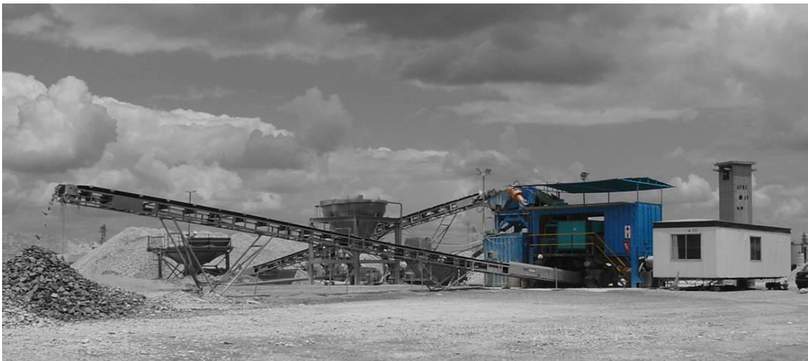
Figure 23. Optical sorter pilot plant at Kloof Gold Mine
