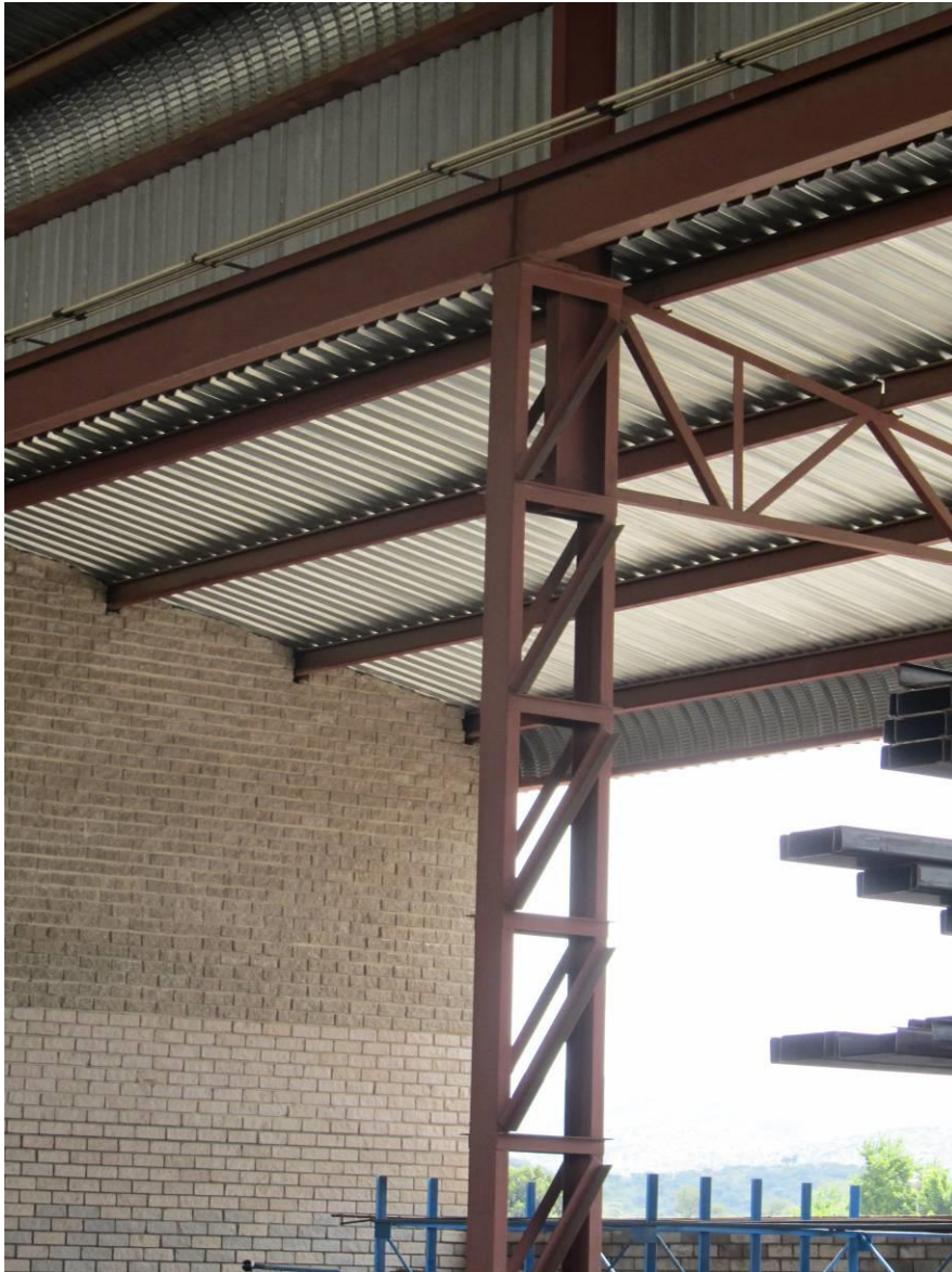
Figure 1:2 Traditional double laced built-up column
