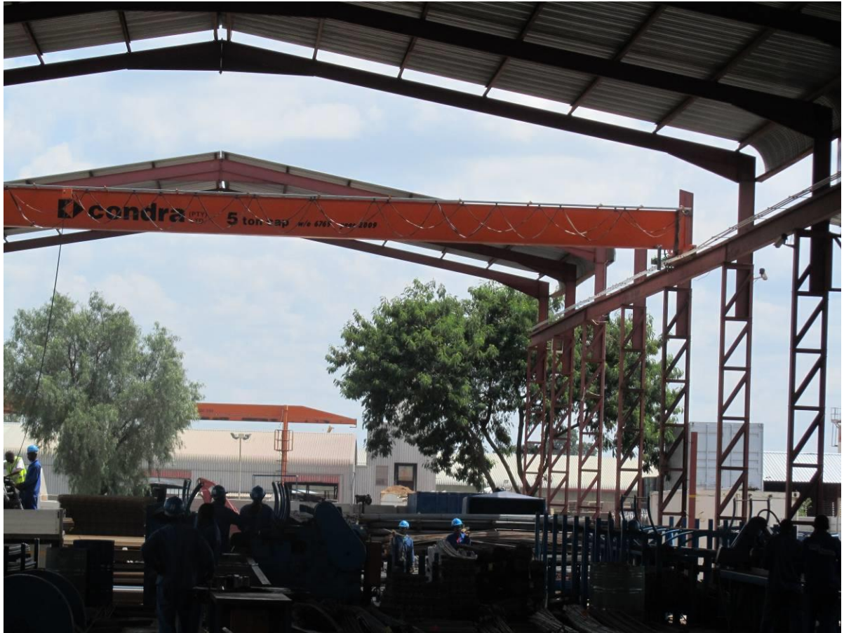
Figure 8:3 Built up column in an industrial ware house supporting crane girder
