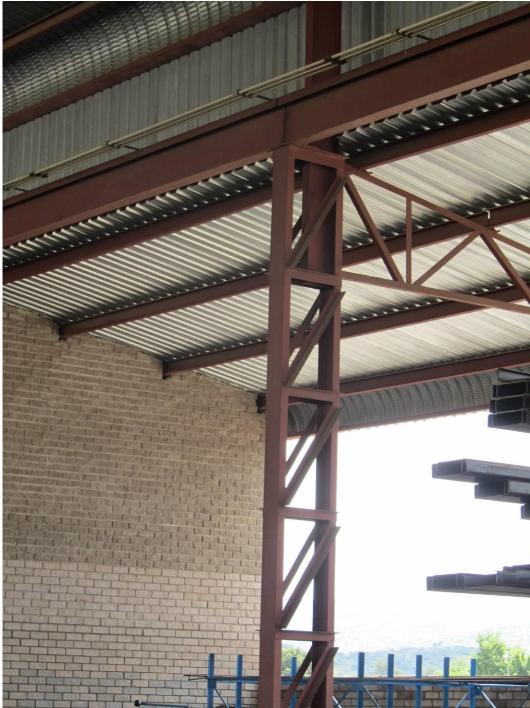
Figure 8:1 Built up column in an industrial ware house
