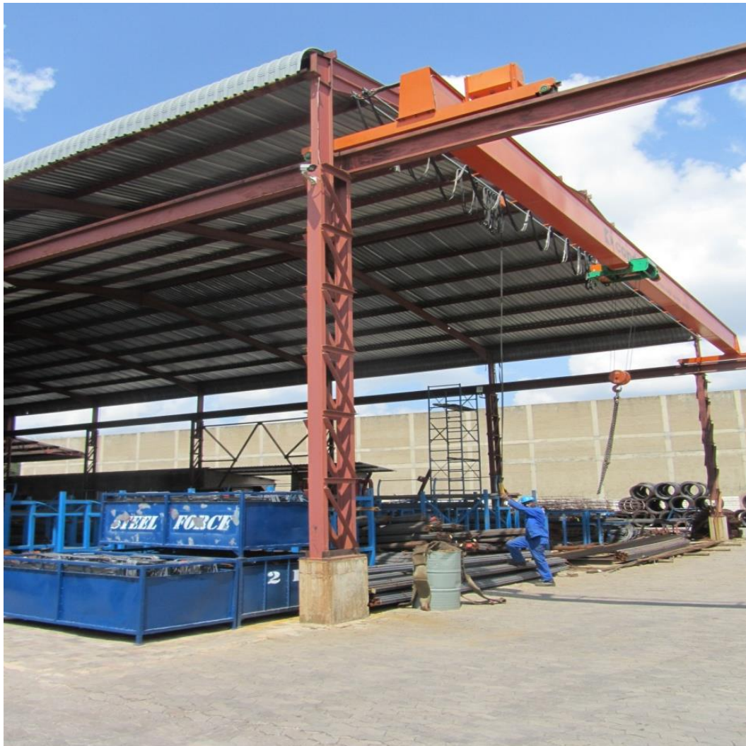
Figure 1:5 Built-up column with lacings in an industrial building
