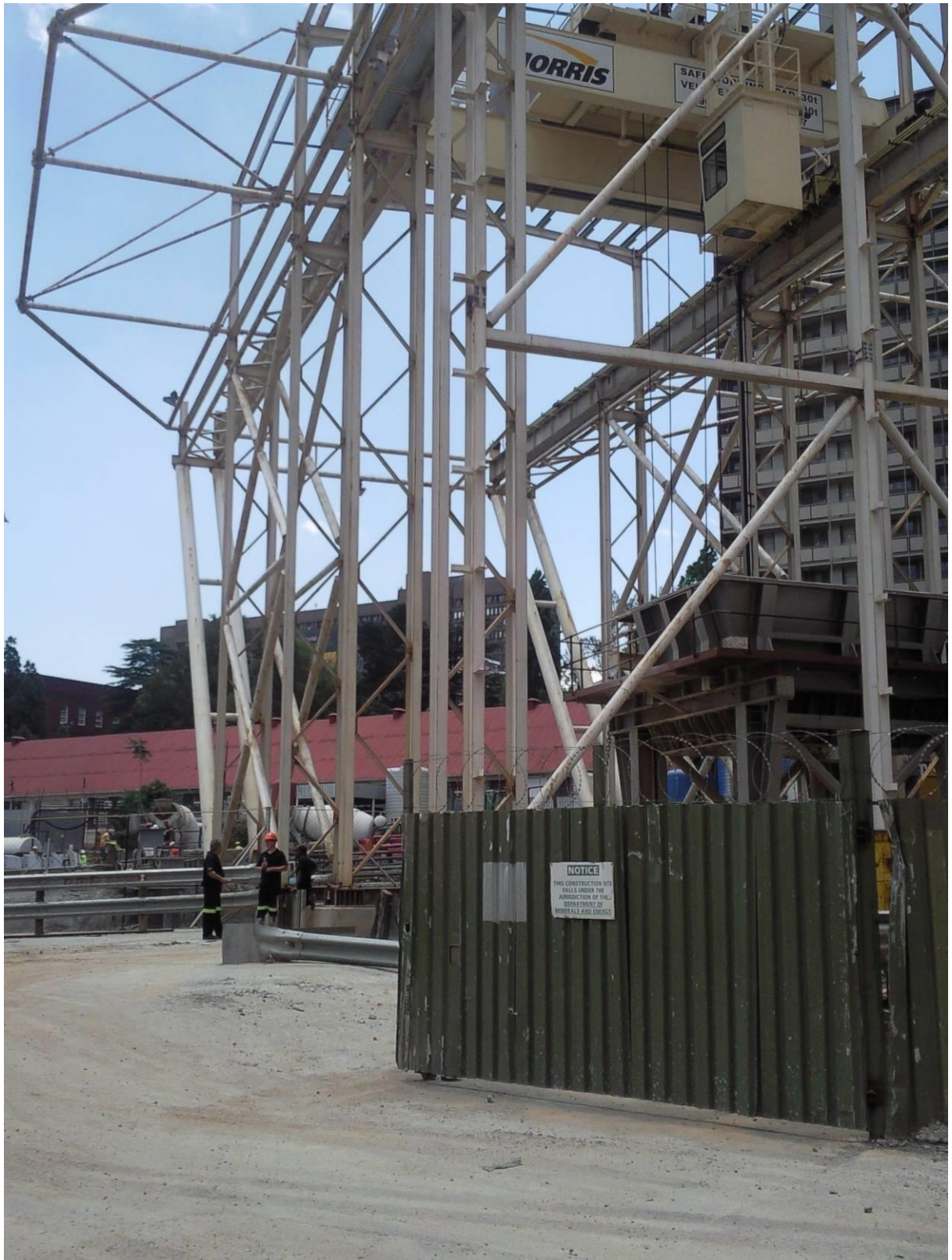
Figure 8:6 Single laced built up column of a crane girder used during Gautrain project
