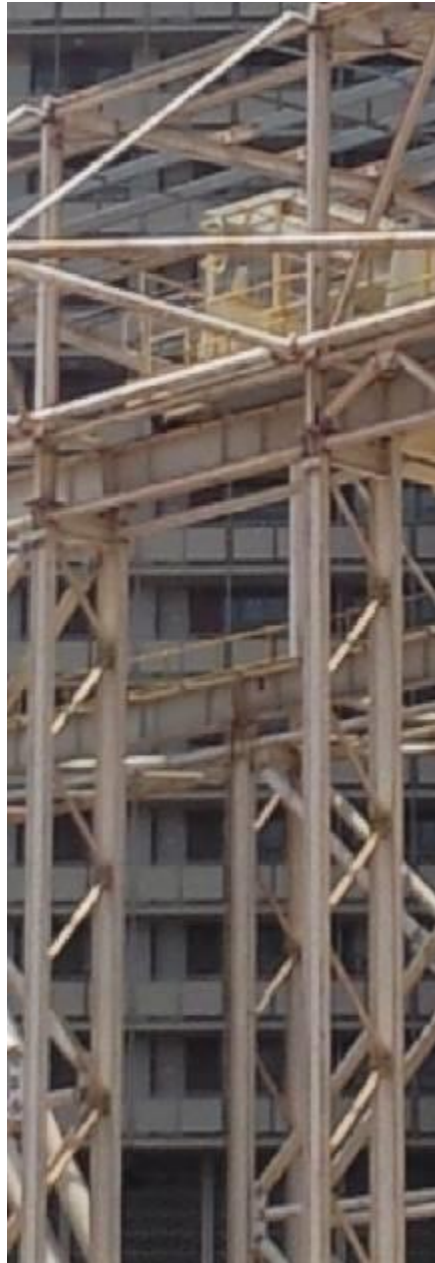
Figure 1:3 Single built-up column
