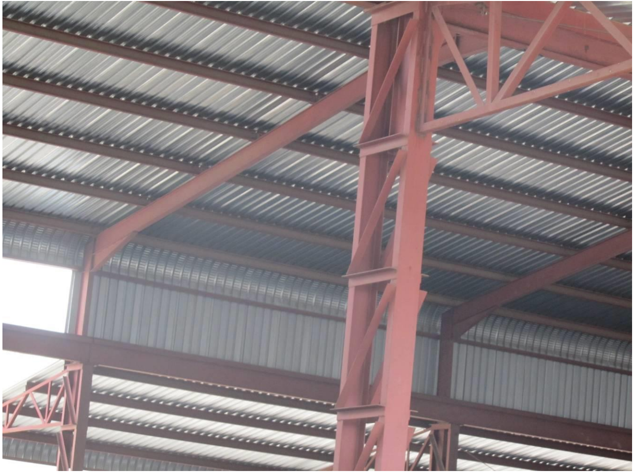
Figure 8:2 Built up column in an industrial ware house supporting crane girder
