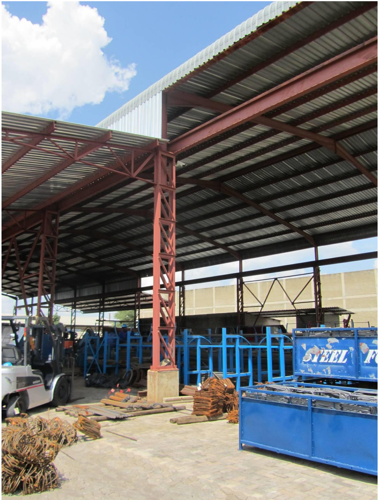
Figure 8:4 Built up column in an industrial ware house supporting crane girder
