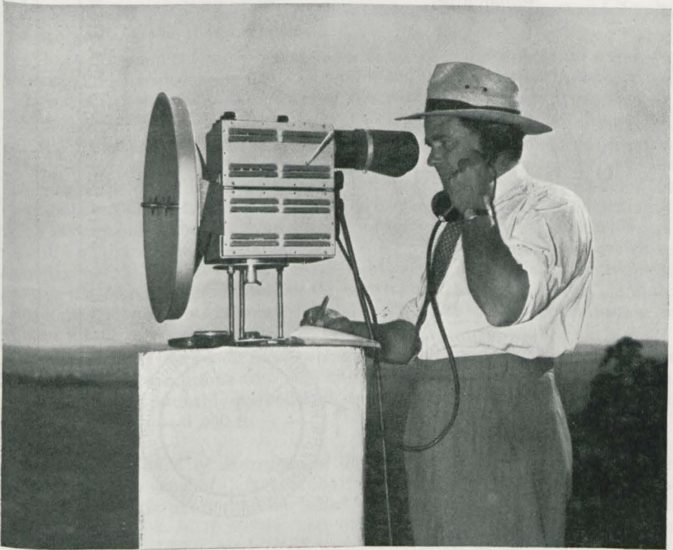
Fig. 1. An experimental model of the Master Tellurometer measuring a line between beacons in Pretoria and Johannesburg.
