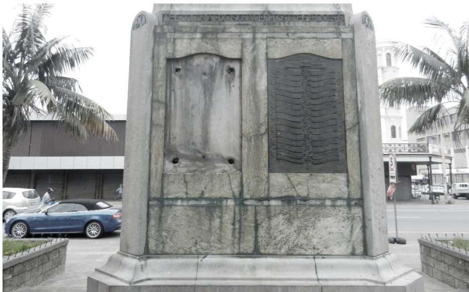
IMAGE 98: Missing plaque at the base of the Colonial Division Memorial (Ndzingani 2021)
