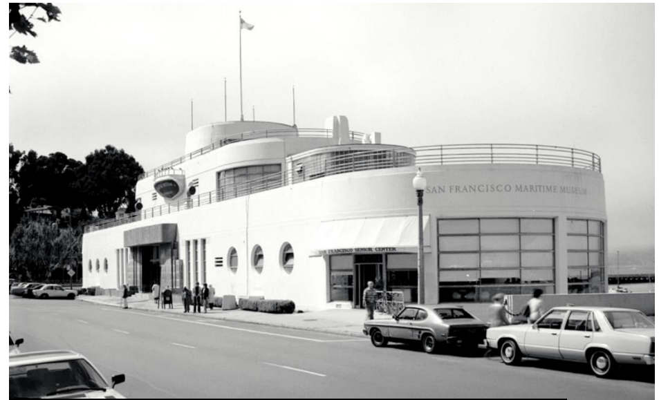
IMAGE 146: General view, rear and side of Aquatic Park Bathhouse (Croteau 1933)
