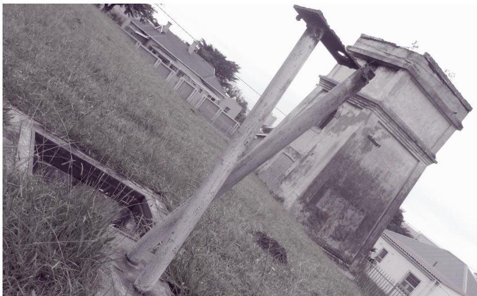
IMAGE 197: Existing manhole of Reservoir Tank (Ndzingani 2020)
