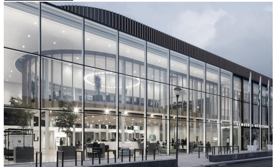
IMAGE 149: An external view of the Council Chamber unit structure above (Van der Wee 2017)
