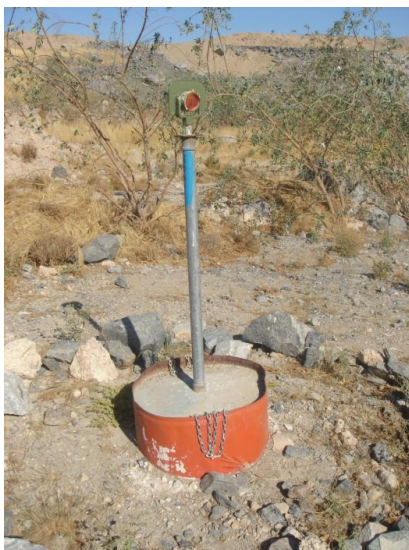
Plate 27 - Mobile slope monitoring point
