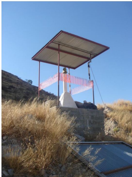
Plate 5 - Erected safety barriers inadequate to prevent injury from falling
