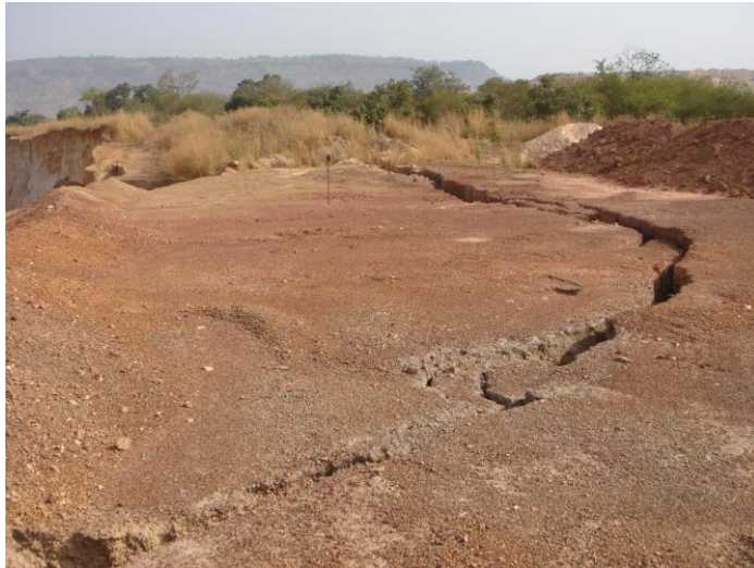
Plate 32 - Tension crack
