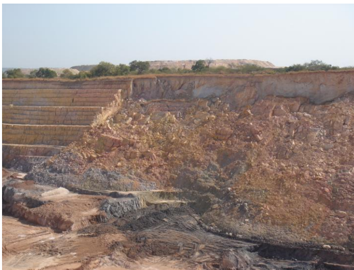
Plate 34 - Composite failure (mix of failure mechanisms - rock mass/circular failure)
