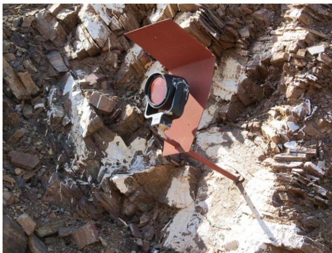
Plate 29 - Face prism for slope stability monitoring with protective cover
