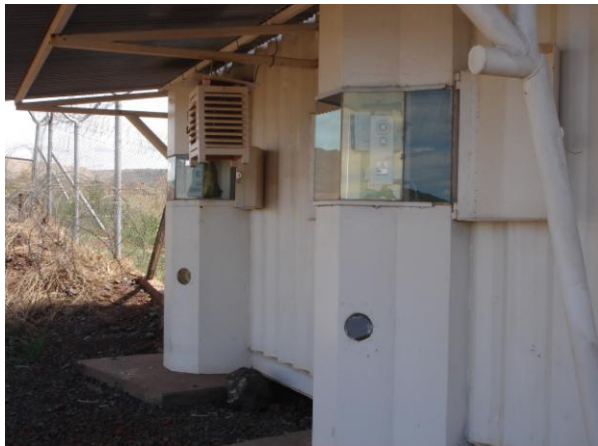
Plate 12 - Slope stability monitoring instrumentation in converted shipping container
