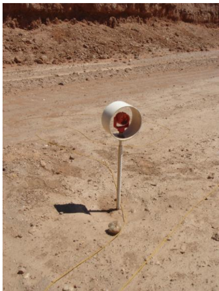
Plate 15 - Bench crest type monitoring point with protective shield for the prism
