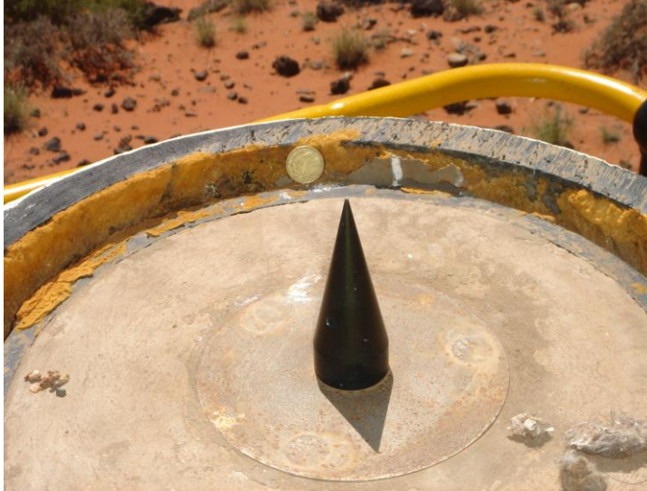
Plate 9 - Plastic outer sleeve of beacon forced up out of concrete base
