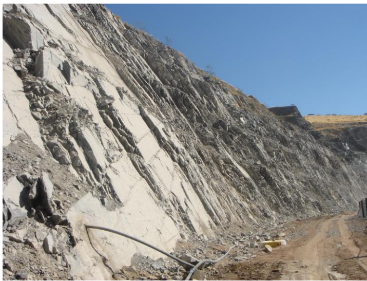
Plate 30 - Planar failure
