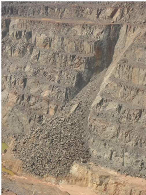
Plate 36 - Wedge failure
