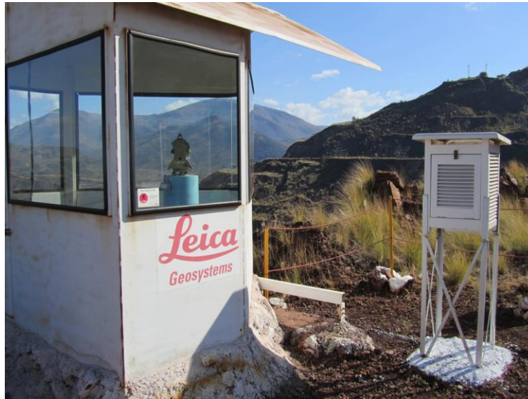
Plate 19 - Transfer beacon in protective shelter with Stevenson Screen for the meteorological sensor
