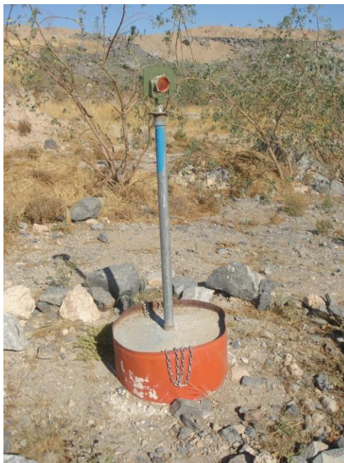
Plate 17 - Mobile type monitoring point with heavy base
