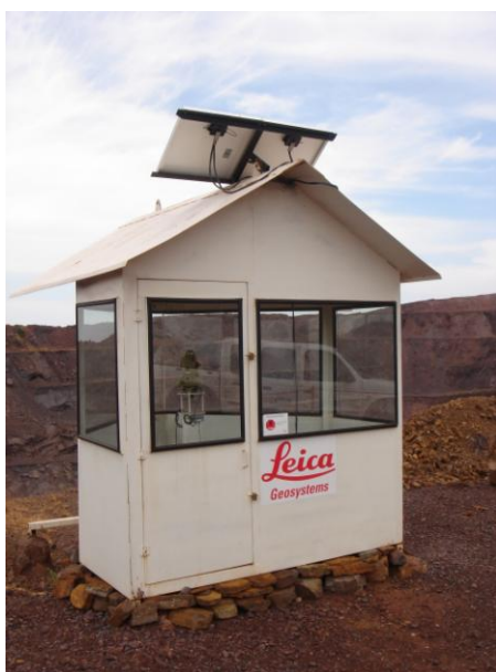
Plate 13 - Slope stability monitoring instrumentation in purpose built protective housing with 360° field of vision
