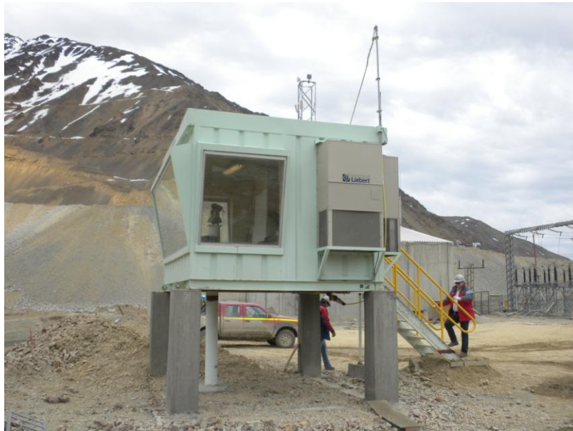
Plate 2 - Protective structure for slope monitoring equipment
