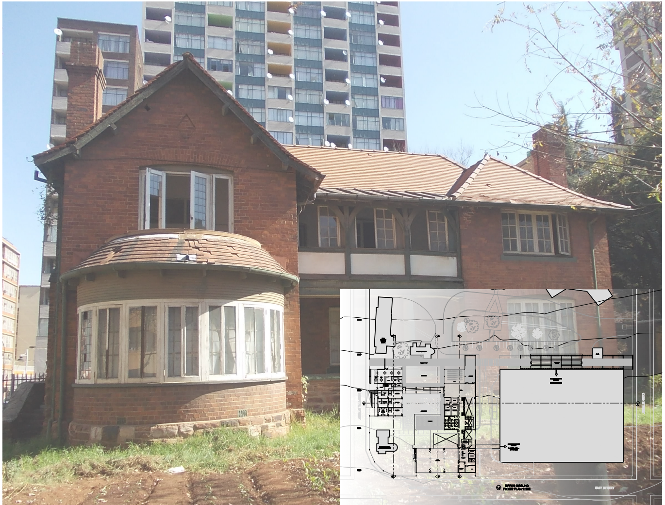
Fig. 51. East elevation of former superintendent's house (Author, 2013)
