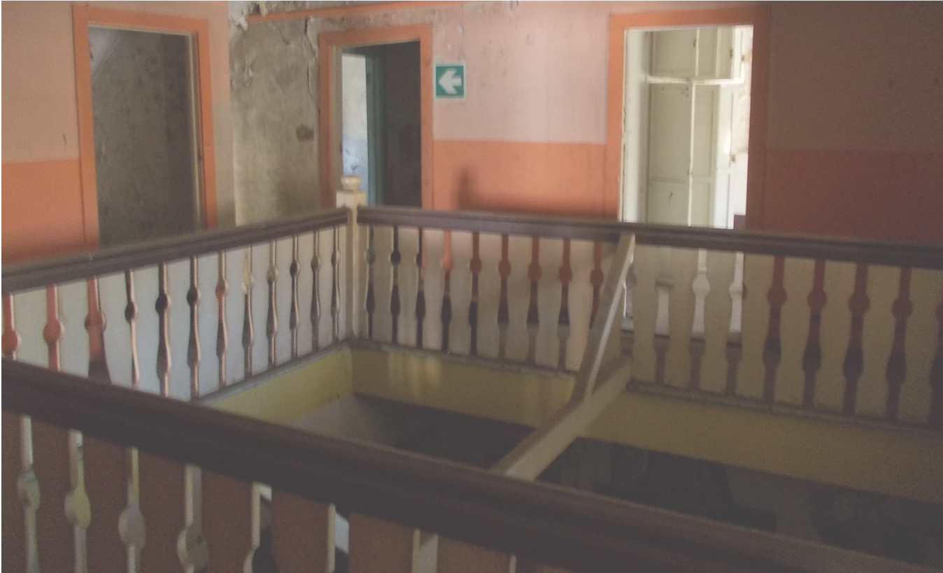
Fig. 53. Double volume inside superintendant's house (Author, 2013)
