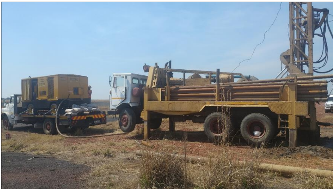
Figure 4-1: Drilling in progress for borehole 1 (BH01).
