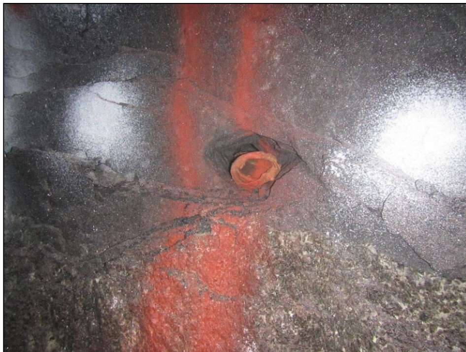
Figure 4.5: A blast socket taken in a panel mining towards south-east
