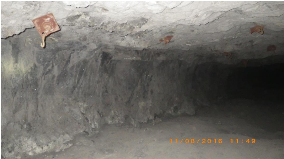
Figure 5.6: A photo of the pillar cut in 15-27 5E panel
