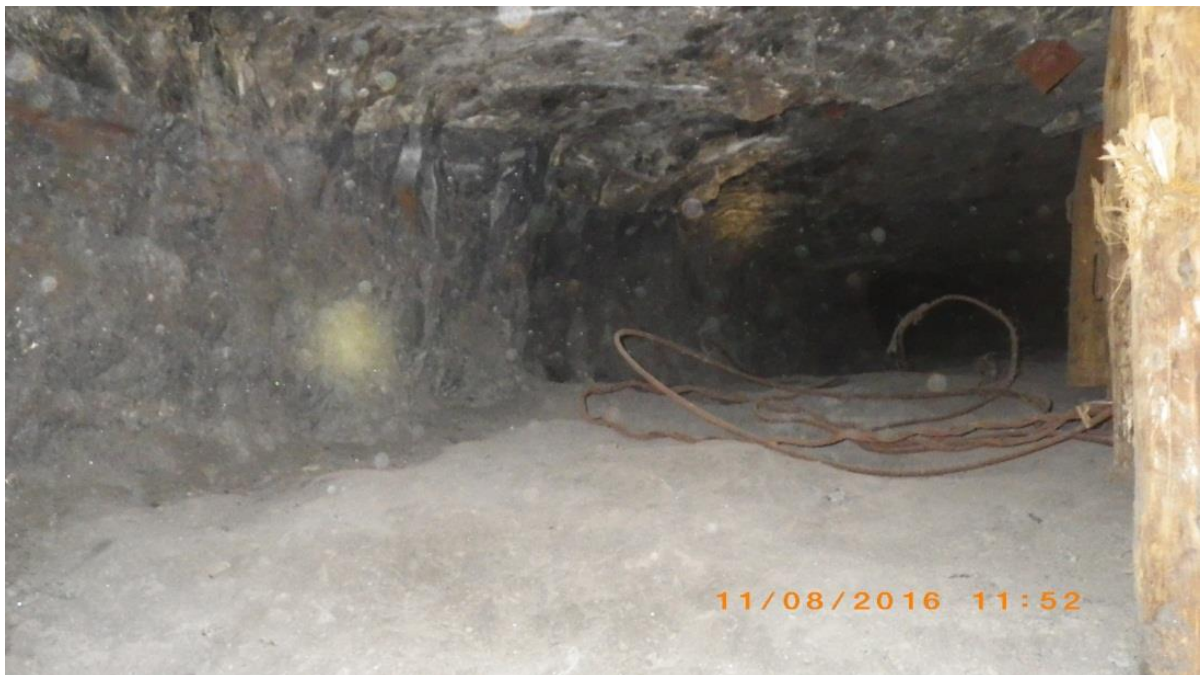
Figure 5.7: A photo of the pillar cut in 15-27 6E panel
