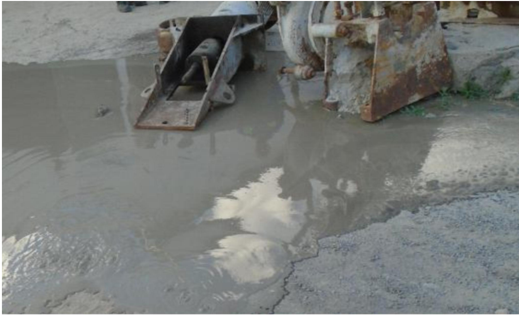
Figure 4.3 Leaks in the process plant
