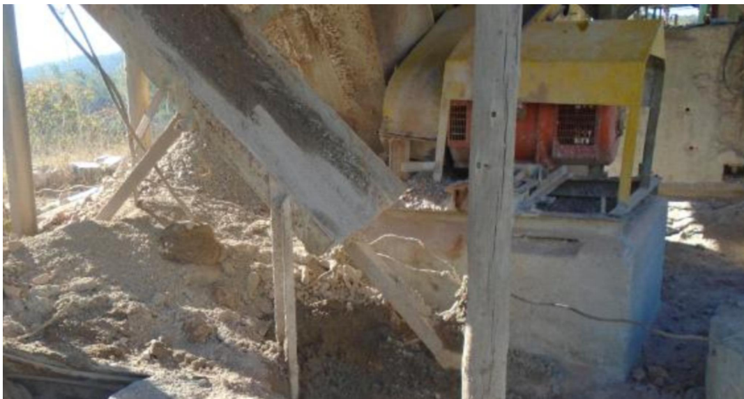
Figure 4.2 Fines spillage in the plant
