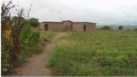
Image 1: Sunnyside High Toilets
