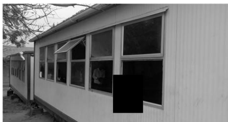
Picture 1: Malcolm Sec Pre-Fabrication Classroom
