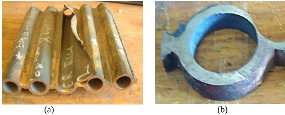
Figure A.3: Failed tubes on division wall of Unit 2 boiler from station A.
