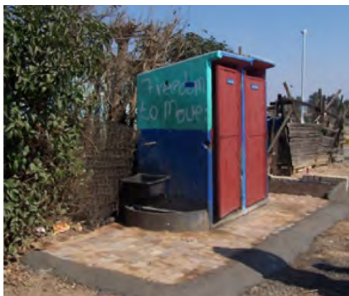
Figure 4.13: Graded brick paving around the toilet block with a small agricultural drain to prevent waterlogging (photograph of point 3b in Figure 4.10)
