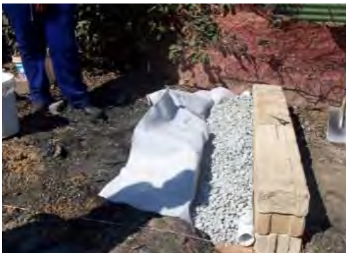
Figure 3.19: Constructed agricultural drain in Diepsloot
