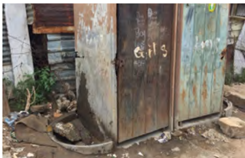
Figure 4.8: Blocked snaking pipe before the intervention (photograph of point 4a in Figure 4.6)
