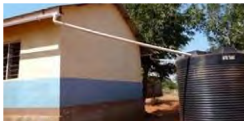
Figure 3.27: Rainwater tank connected to a communal building drainage outlet
