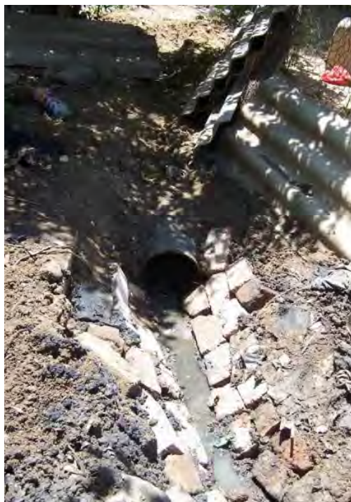
Figure 4.8: Blocked snaking pipe before the intervention (photograph of point 4a in Figure 4.6)
