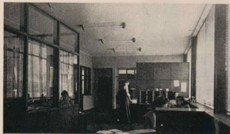
RIGHT, ABOVE: The west elevation of the Office Block showing the main entrance porch. The Venetian blinds provide sun control for the main office windows. BELOW: Interior of the general office seen from the public space at the entrance.
