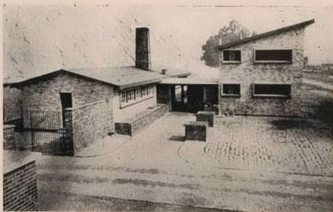
The Hostel group seen from the upper landing of the Manager's Flat.
