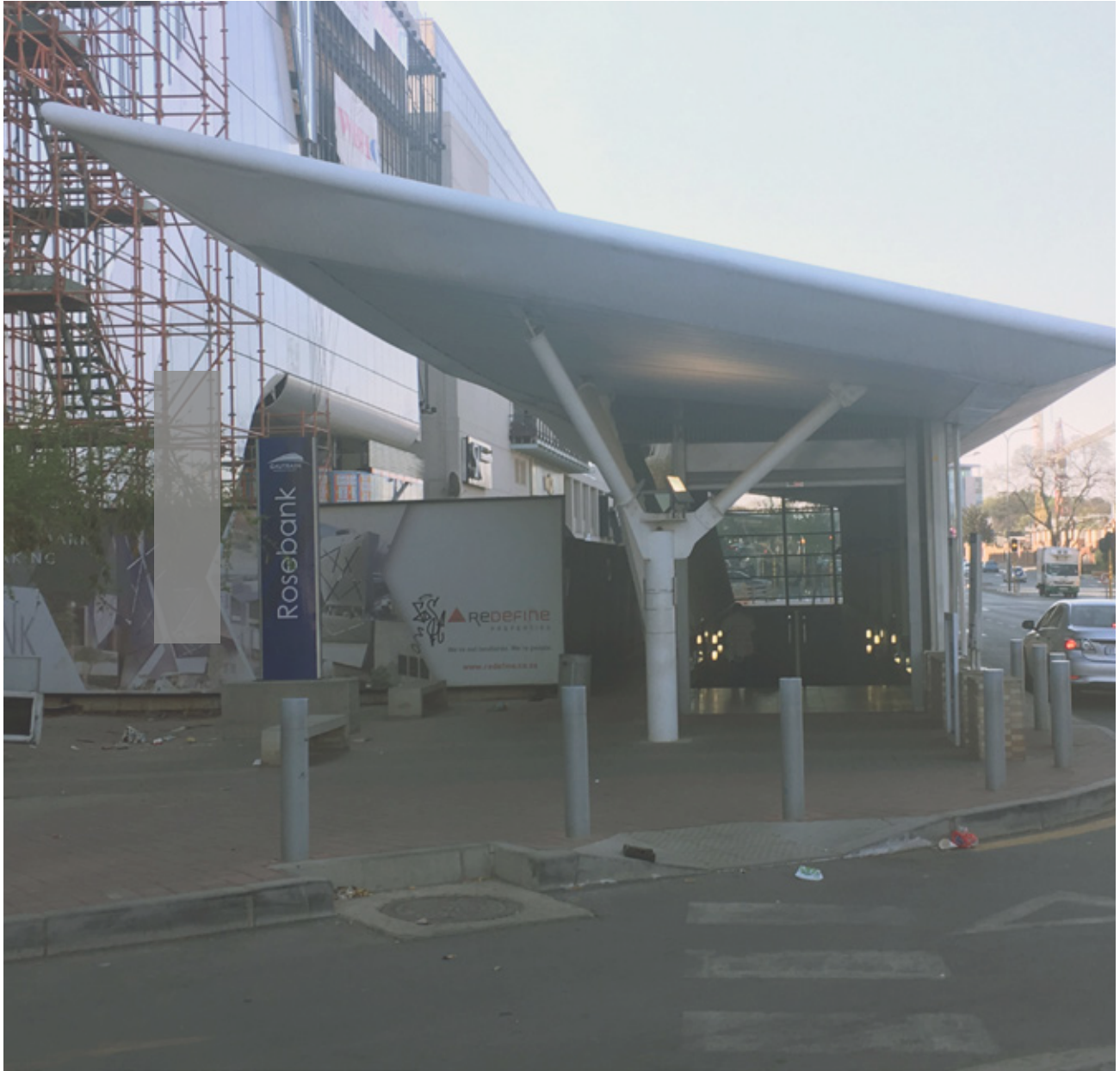
Figure: 4.8 - Gautrain Pedestrian Entrance The implementation of Gautrain resulted in Rosebank becoming a transportation node with various levels of transit available to the public.
