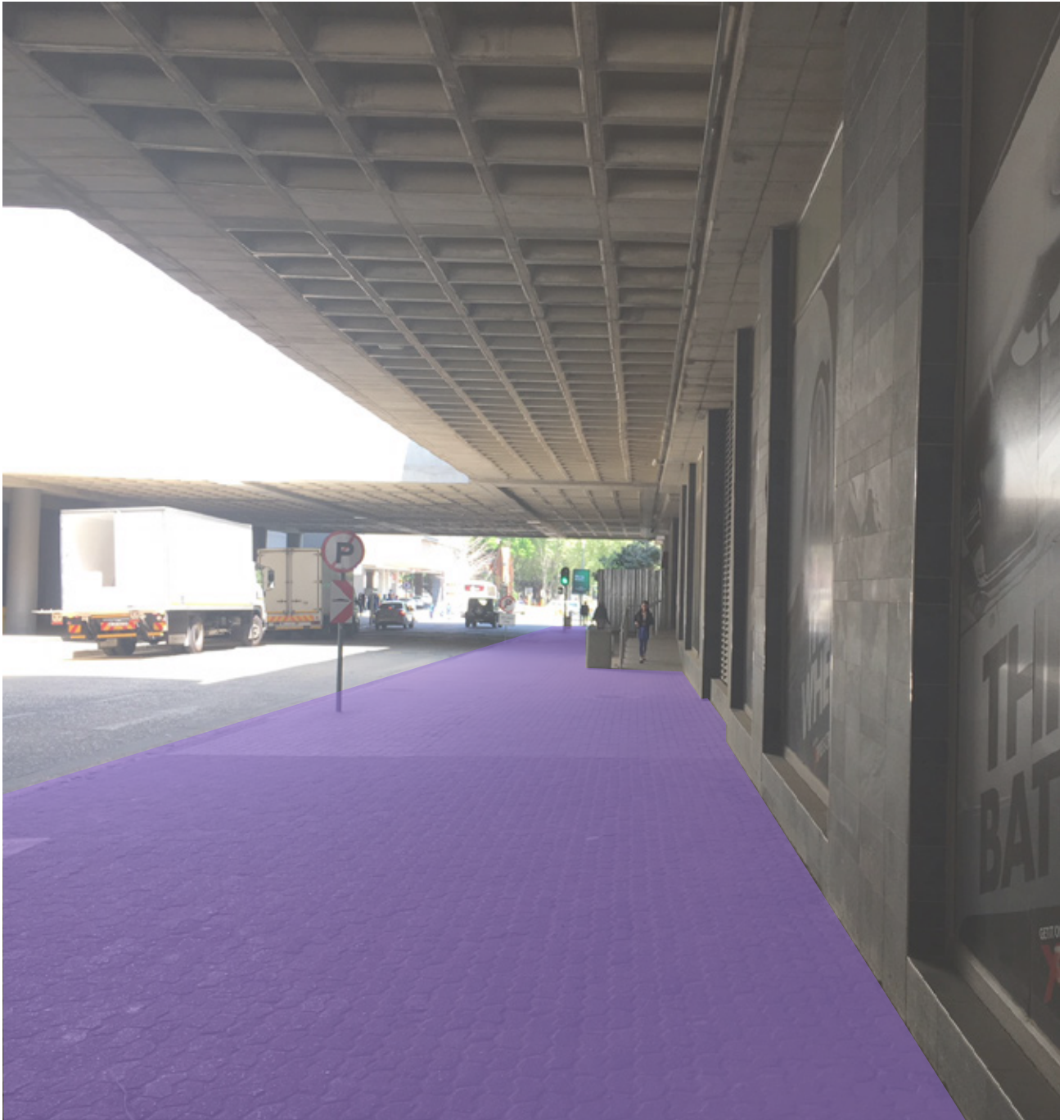
Figure: 4.17 - Sidewalk Under Mall Bridge Wide sidewalk denotes a pedestrian orientated plane, however, the limited light and harsh treatment has resulted in a cold environment resulting in limited pedestrian movement along Bath Avenue
