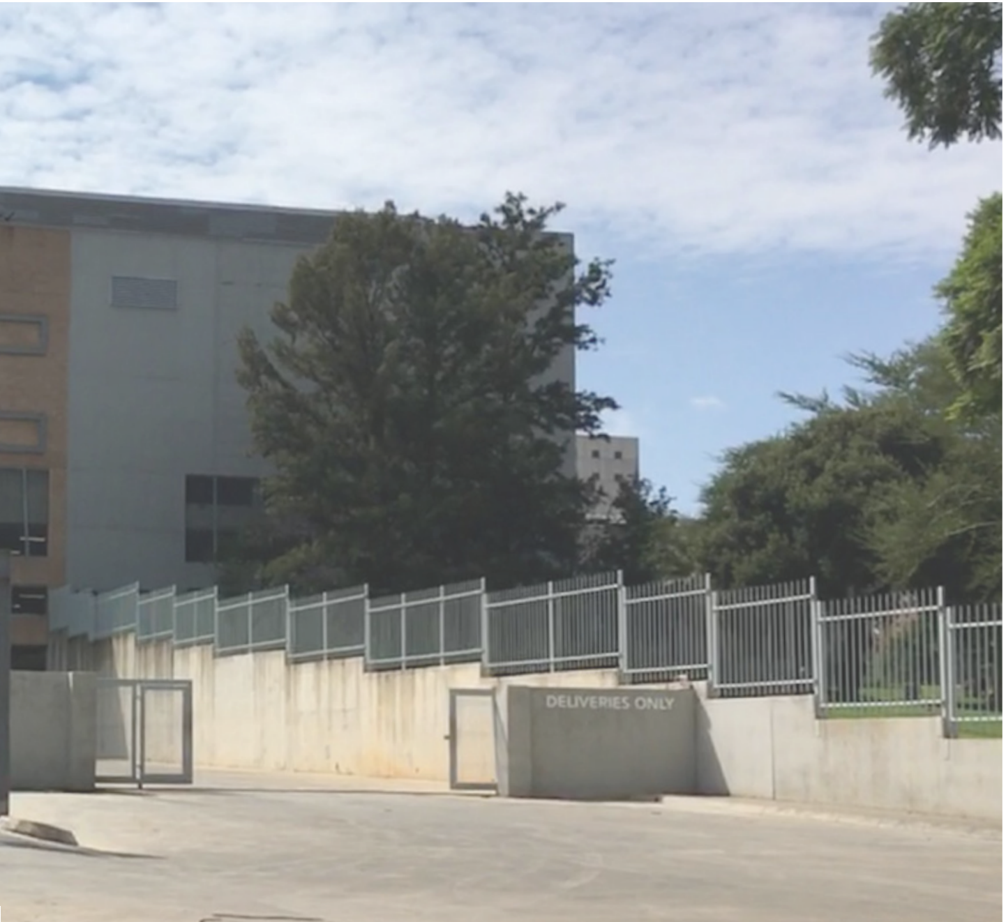
Figure: 4.24 - Parking Garage Sturdee Ave Entrance
